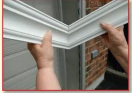
Create perfectly fitting interior crown molding joints
