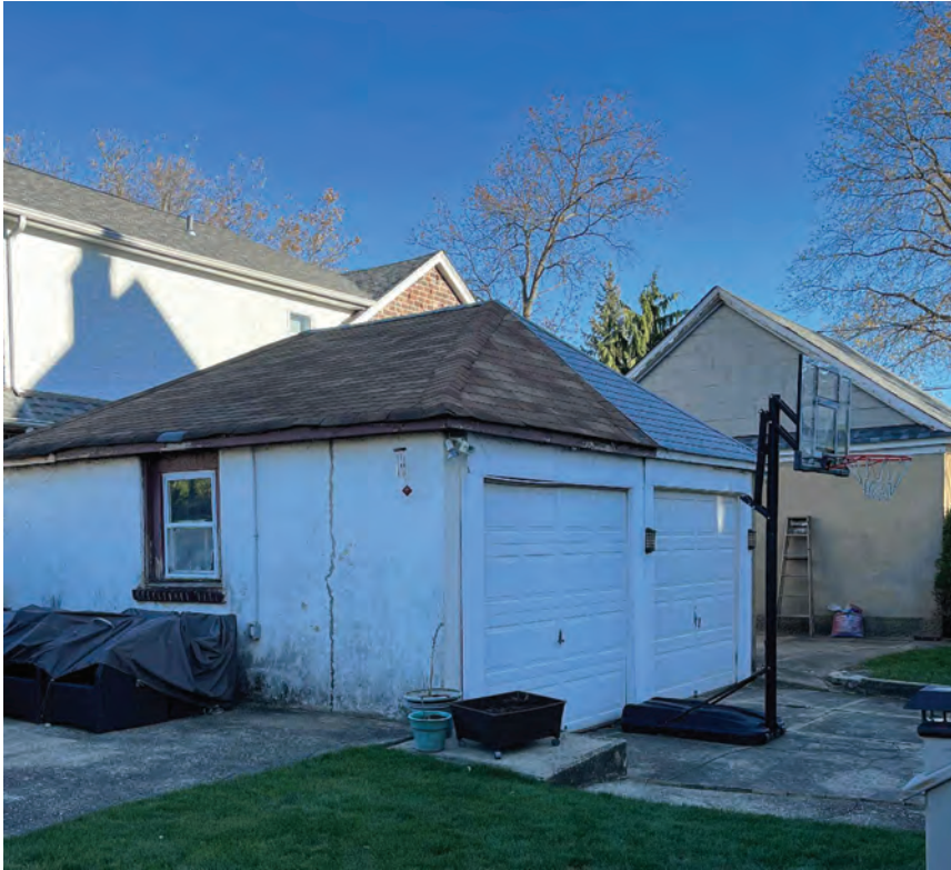
EXISTING SHARED GARAGE TO BE DEMOLISHED
