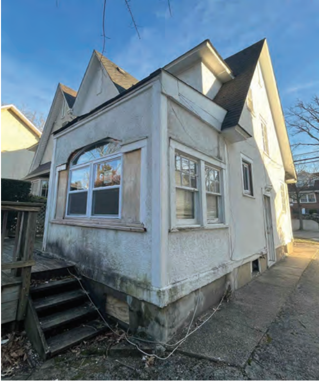
SUN ROOM- N-W
