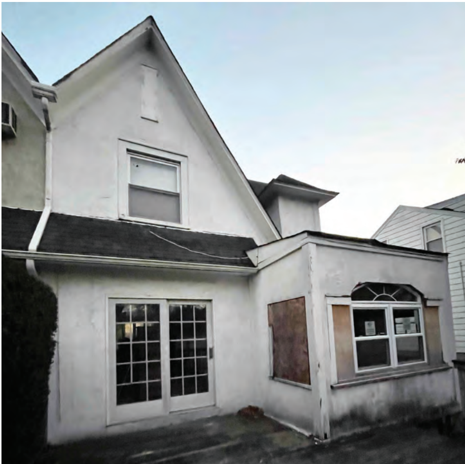
RIGHT SIDE VIEW- WEST
