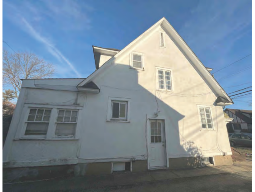
WEST SIDE VIEW " DRIVEWAY"
