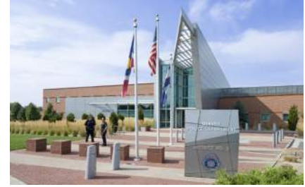
City of Denver Substations 1, 2 and 3 Denver, CO
