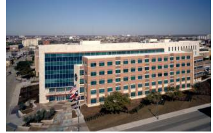
Jack Evans Police Headquarters Dallas, TX
