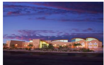
Glendale Public Safety Building Glendale, AZ
