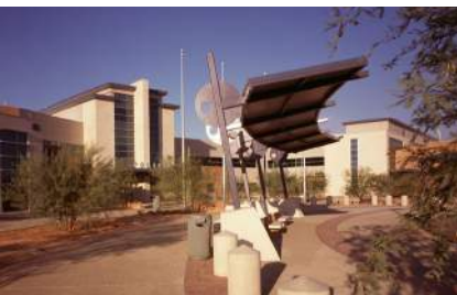
Town of Gilbert Public Safety Building · Gilbert, AZ
