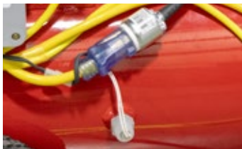
Low fluid heater cutoff float switch
