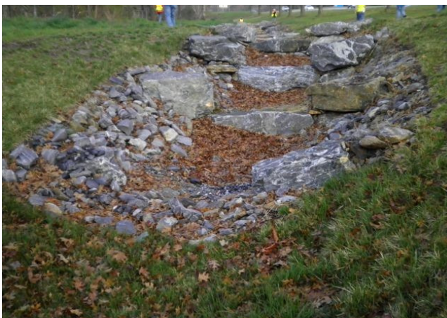
Biofiltration conveyance system installed in an NCDOT ROW
