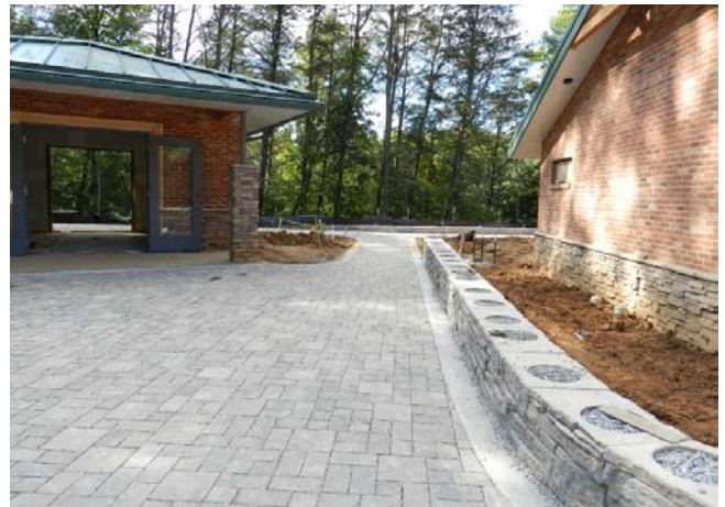
Permeable pavers installed at a rest area
