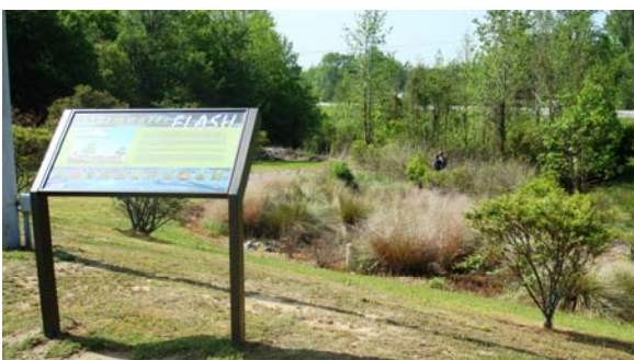
Bioretention basin and public educational display at a NCDOT rest area
