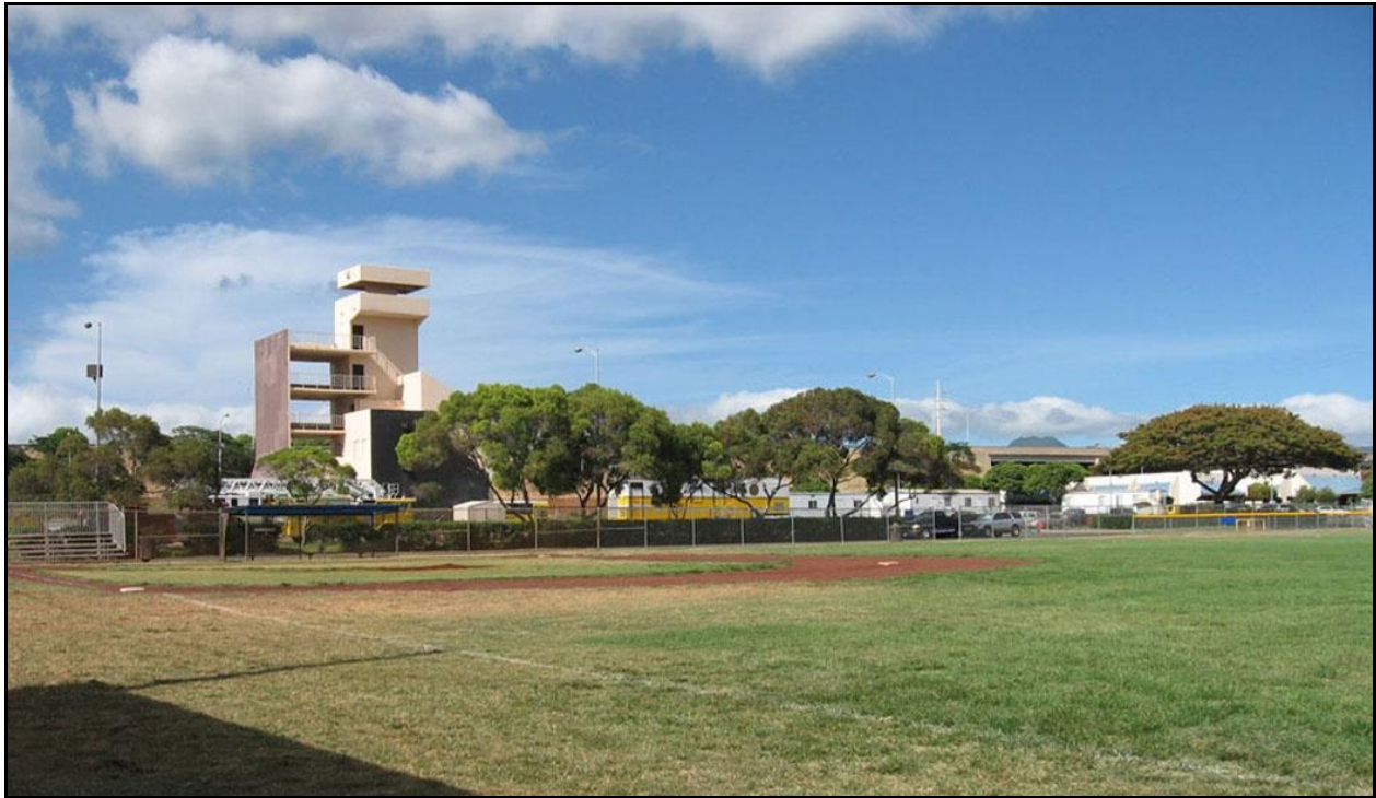
Figure 3-17 Existing view of the Training Center looking mauka from Lynch Park (Key 5)
