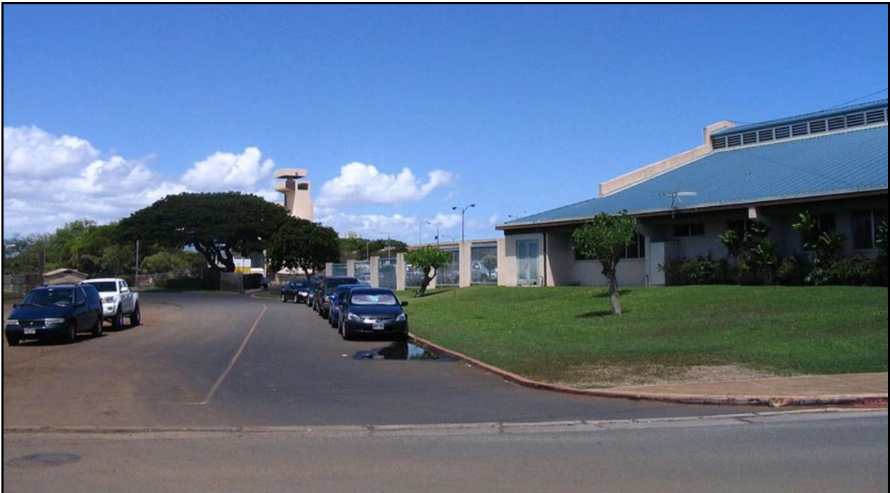
Figure 3-16 Existing view of Mokulele Fire Station on the corner of Paine Circle and Valkenburgh Street (Key 4)
