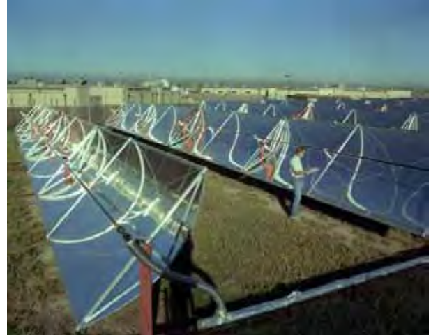
Figure 3.17. Parabolic trough collectors used to heat water at a large prison facility in Colorado.
