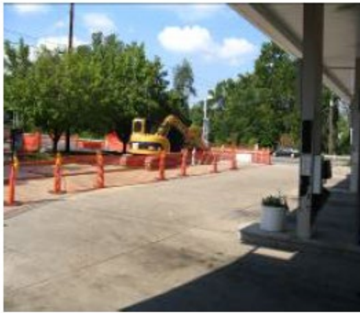
Example of Level 2 Traffic Control
