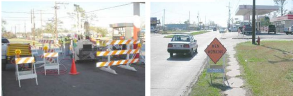
Examples of Level 2 Traffic Control
