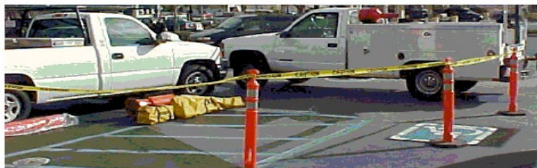
Figures A1.2.2(a)(b)(c) - Examples of Level 2 Traffic Control
