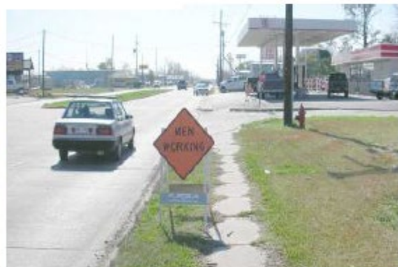
Example of Level 2 Traffic Control
