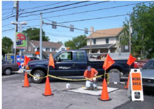
Example of Level 1 Traffic Control
