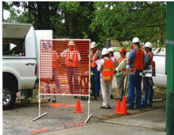
Barrier constructed of PVC pipe and orange fencing
