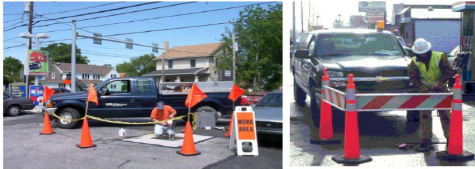
Figures A1.2.2(a)(b)(c) - Examples of Level 2 Traffic Control
