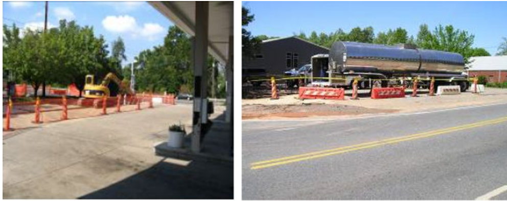
Examples of Level 2 Traffic Control
