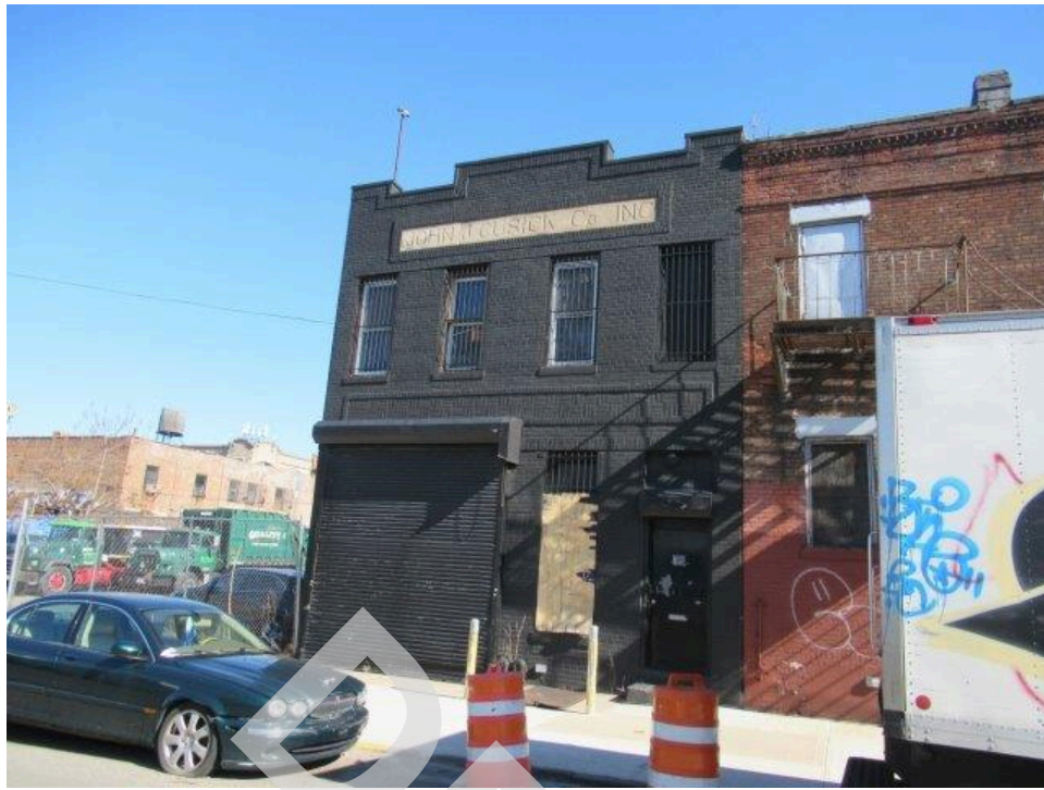
1. View of the south elevation of subject building
