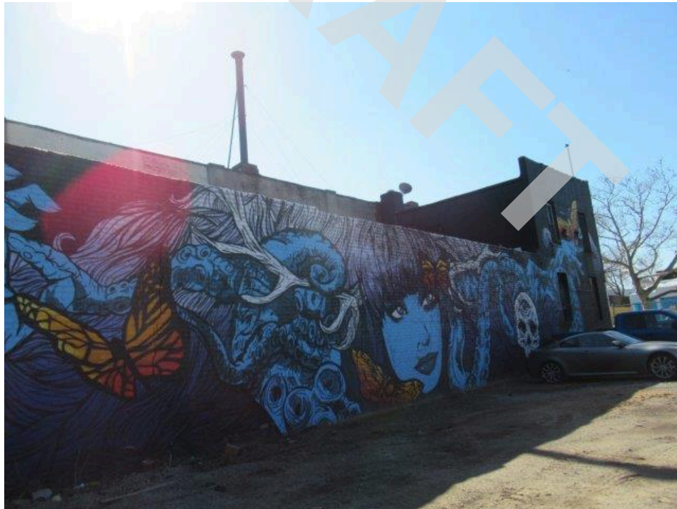
2. View of west elevation of subject building
