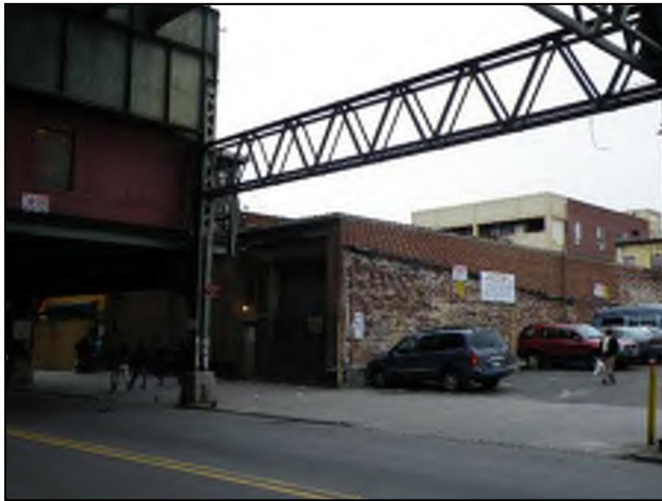
Eastern adjoining NY Transit Substation
