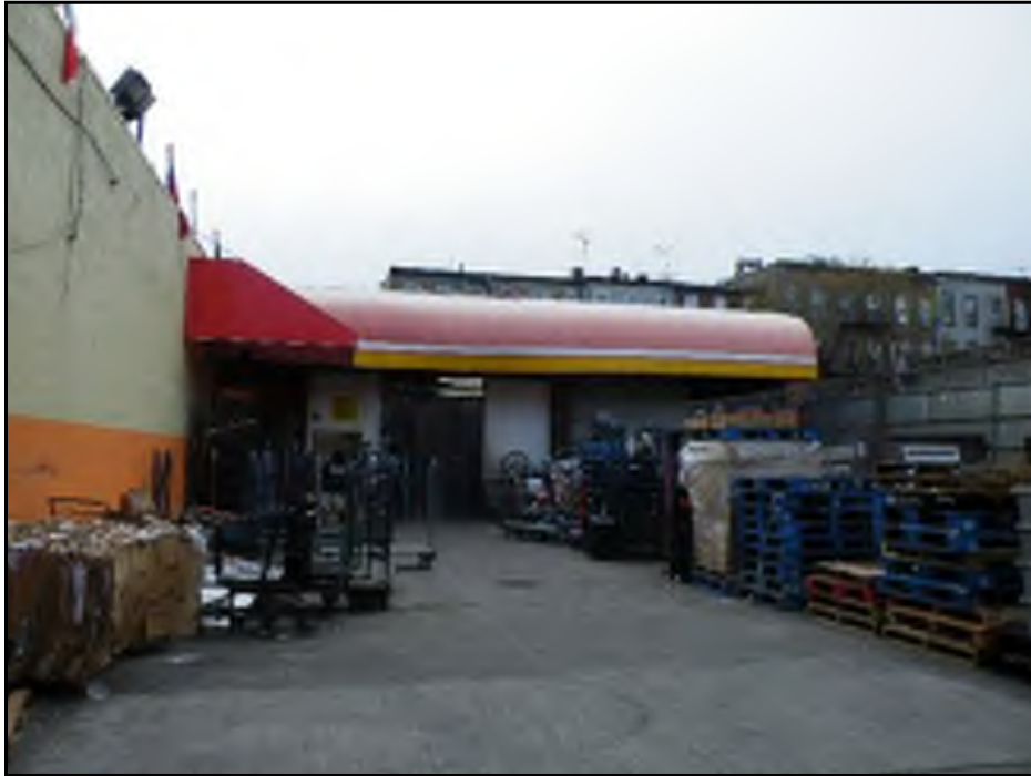
Warehouse addition on western side of building
