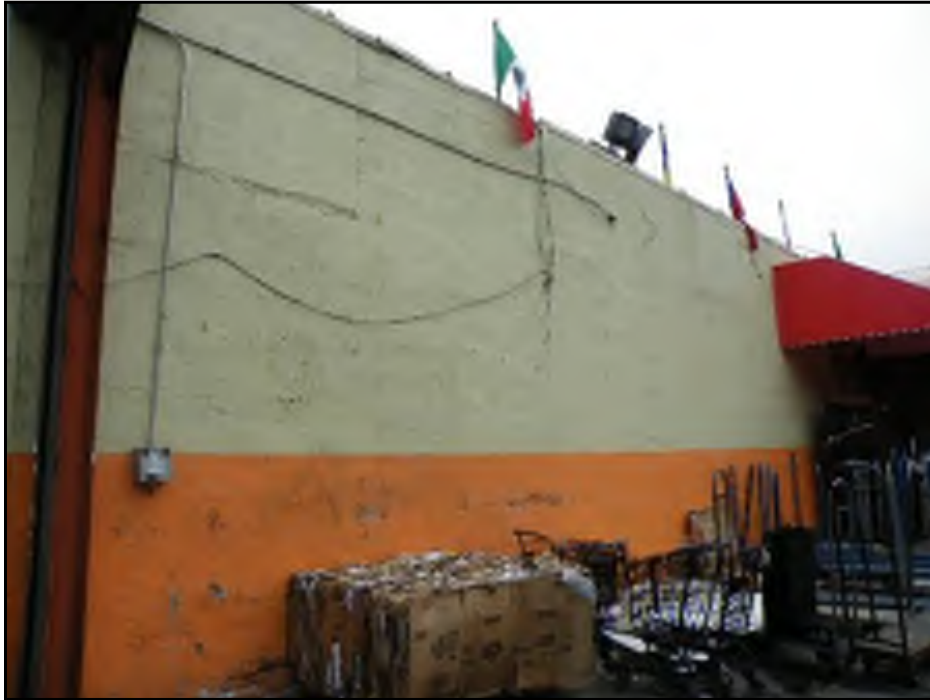
Western exterior wall (loading dock)
