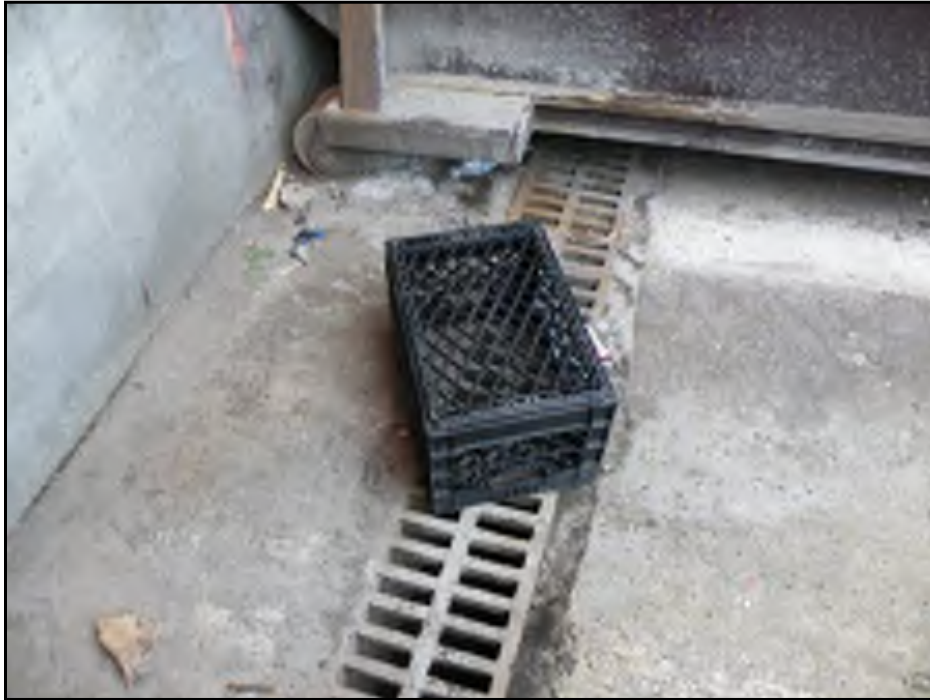
Trench drain in loading dock area
