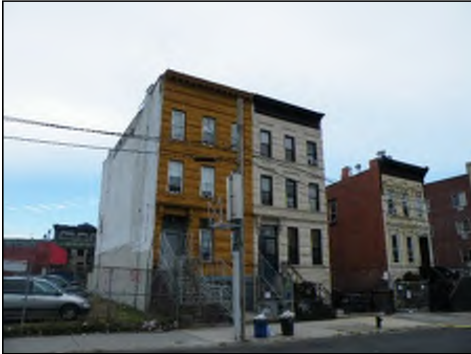
Southern adjoining residential dwellings
