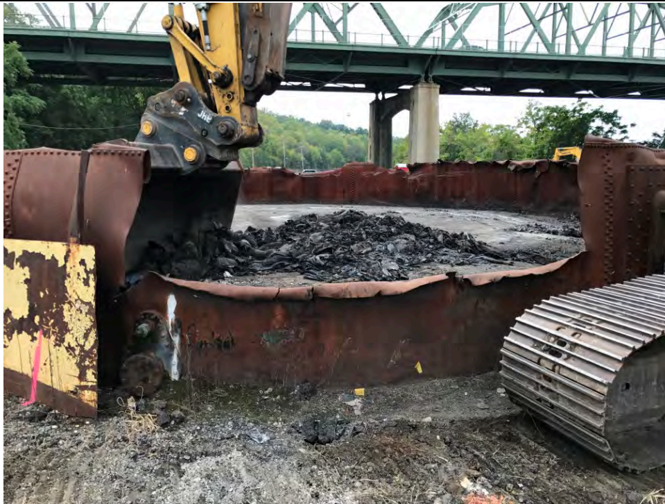
Date: 09/21/2017 Site Name: Troy (Water Street) Site - Area 3 Photographer's Initials: JAJ Description: Photograph #12: Tar material scraped off concrete within Former Tank T-41. Photograph taken facing South.
