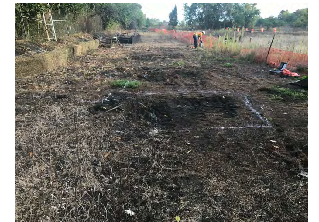
Date: 09/20/2017 Site Name: Troy (Water Street) Site - Area 3 Photographer's Initials: JAJ Description: Photograph #4: Erosion control measures (hay bales and silt fence). Photograph taken facing North.
