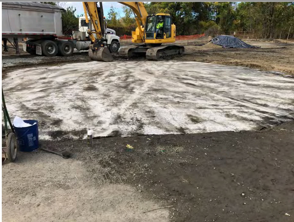
Date: 10/16/2017 Site Name: Troy (Water Street) Site - Area 3 Photographer's Initials: JAJ Description: Photograph #18: Concrete pad beneath Former Tank T-41 after completion of excavation of overlying soils. Photograph taken facing Northwest.
