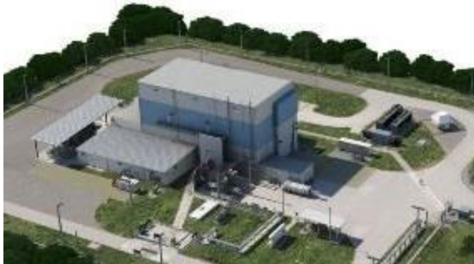
Figure 7-4. Multi Payload Processing Facility (MPPF)
