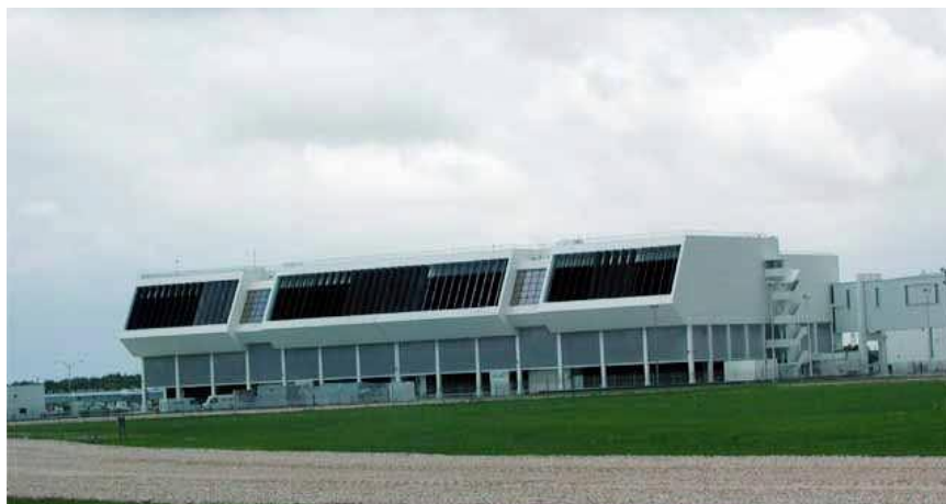
Figure 7-13. Launch Control Center
