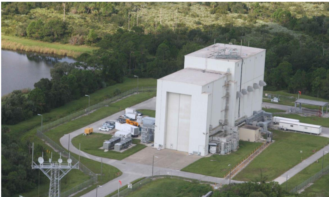
Figure 7-6. Payload Hazardous Servicing Facility (PHSF)
