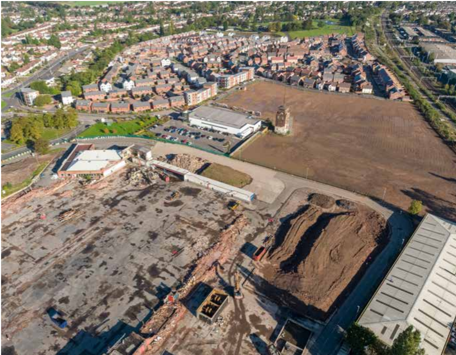
Demolition, remediation, construction and re-occupation of the Goodyear Site
