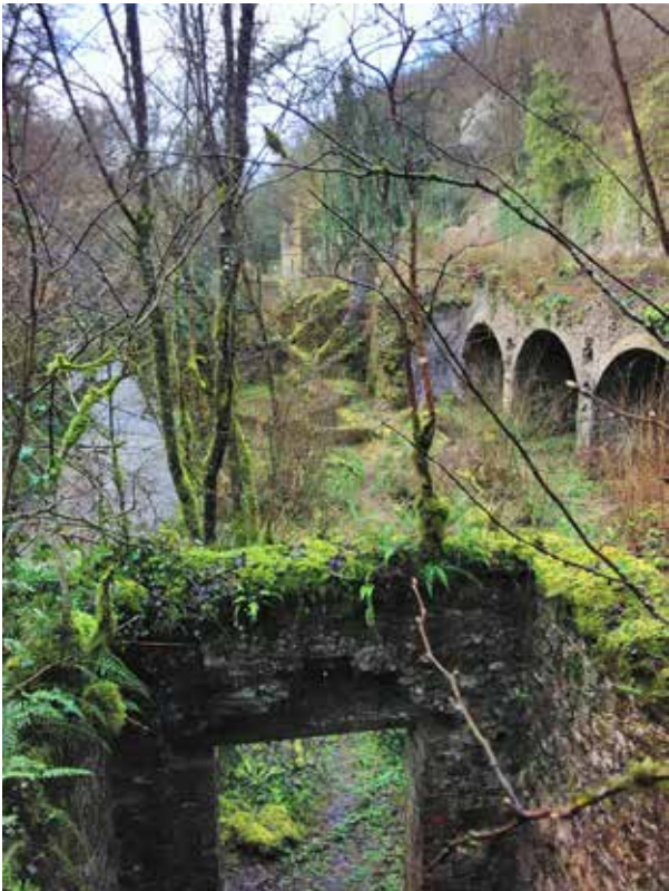
Fussel Iron Works by Will Thorpe, Southwest Environmental Ltd
