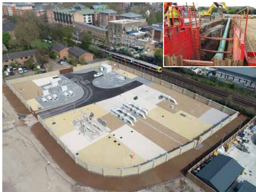
Completed PRS and gas main installation (top right)
