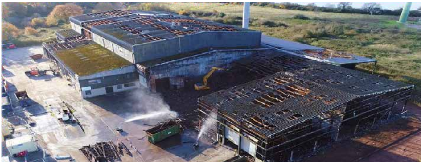
Guillotine breaker deployed at site
