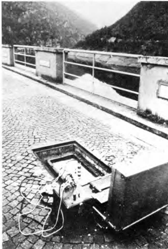
Figure 8. Application of the TLPP method on an Italian concrete dam.
