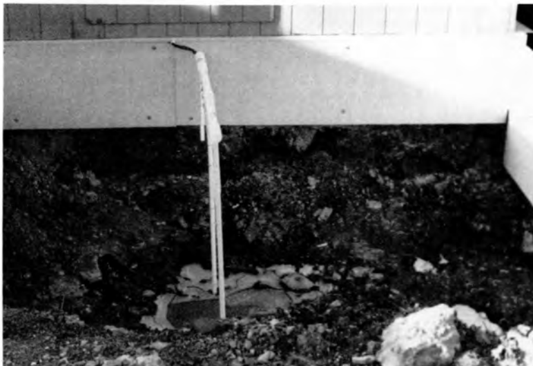
Figure 7. Photos of test insulation installation. (a) Foundation wall with heat-flux transducer plates prior to the insulation installation. (b) Top 0.25-m- (10-in.-wide pieces of XEPS installed. (c) Finished test panel before backfilling.
