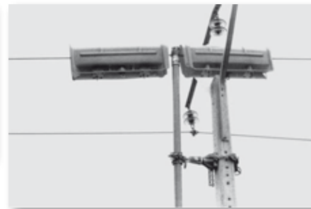
Montage en mât Mast assembly during construction
