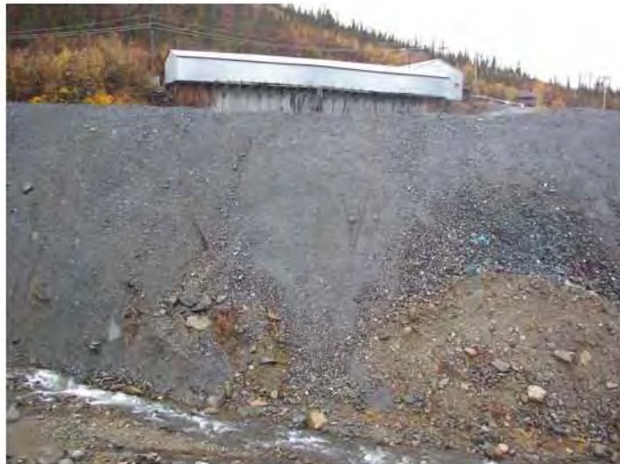
Photos 22.13b_Bellekeno dump toe in creek
