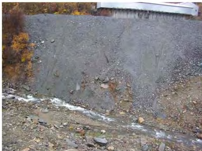
Photos 22.13c_Bellekeno dump toe in creek
