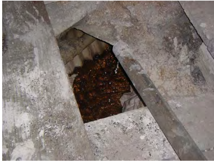
Photo 22.4_Bellekeno lime addition detail
