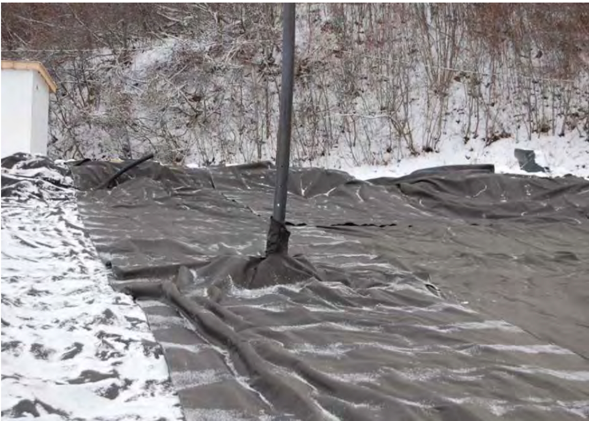
FIGURE 17. GEOTEXTILE PLACEMENT PRIOR TO COVER MATERIAL PLACEMENT.
