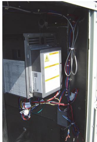
Figure 7. Factory installed VFD assembly
