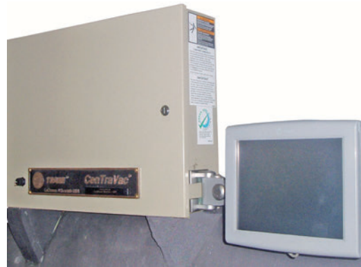
Figure 18. Arm/display assembly mounted at alternate location
