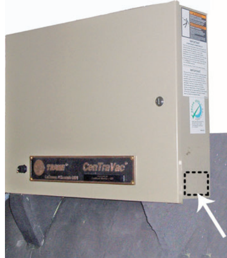
Figure 18. Arm/display assembly mounted at alternate location
