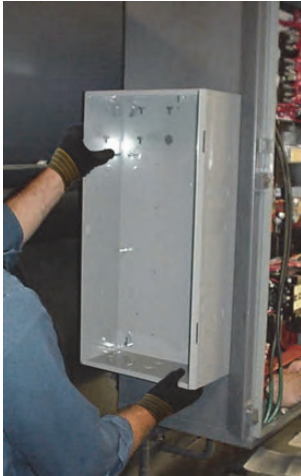
Figure 45. Mounting starter sub-box
