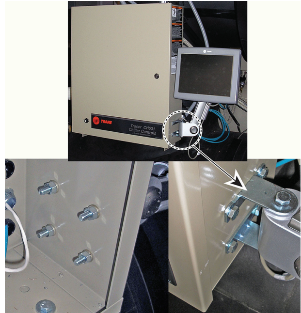
Figure 4. Bolting display arm to the panel
