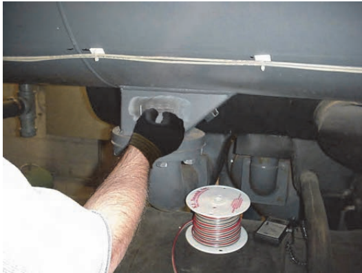
Figure 9. Sensor mounting with Armaflex insulation
