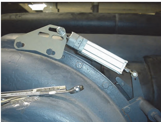
Figure 11. Installed stepper IGV actuator
