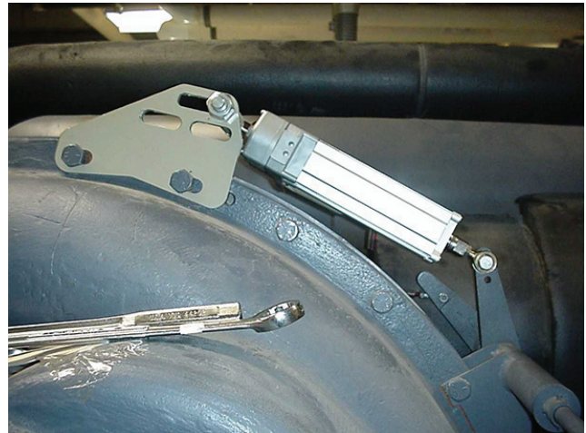
Figure 13. Installed stepper IGV actuator
