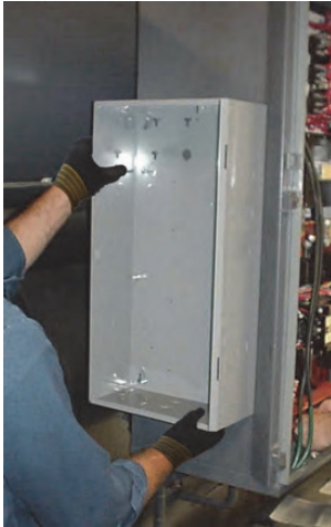
Figure 46. Mounting starter sub-box
