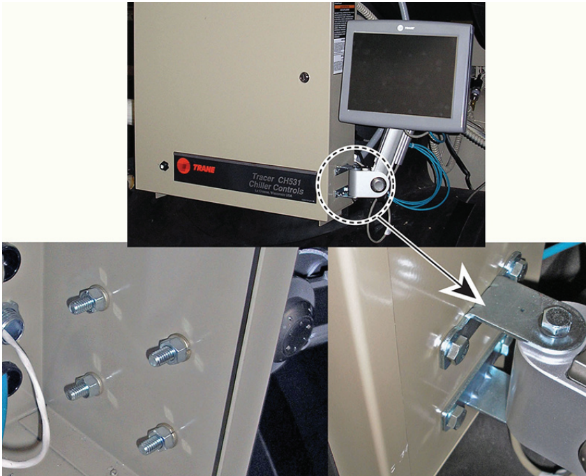
Figure 7. Bolting display arm to the panel
