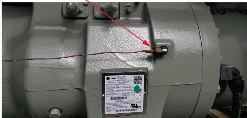
**Figure 15. Intermediate oil pressure transducer location**
