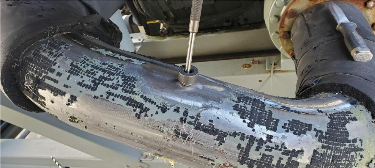
**Figure 20. Follow standard welding procedures when welding 1/4 inch pipe thread threadelet in place**
