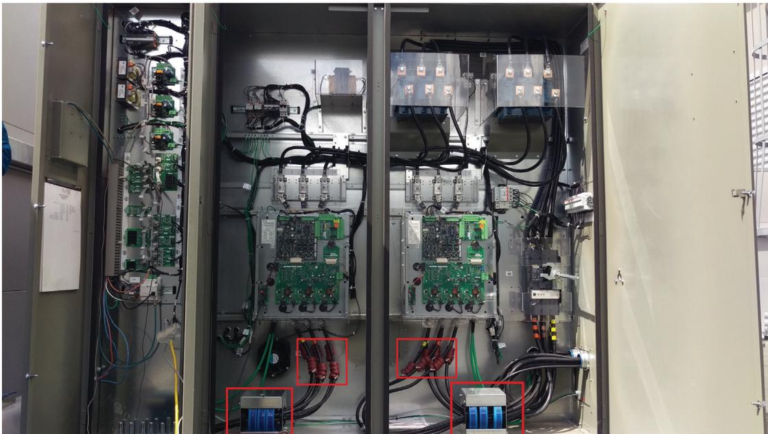
common mode chokes are necessary. The choke assembly encircles all current carrying conductors between the drive and compressor. Do not include ground conductors. Individual cores must also be installed on the power conductors. Refer to the schematic and image below. With removal of the output inductor, the power conductors will be need to be spliced together. Polaris electrical connectors are recommended (Catalog No.: IT-250). Six pieces are needed. There are two conductors per phase.
