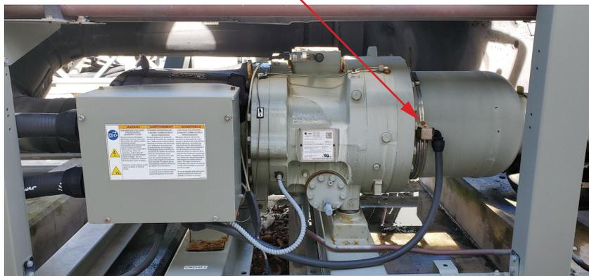
**Figure 14. High pressure switch location**
