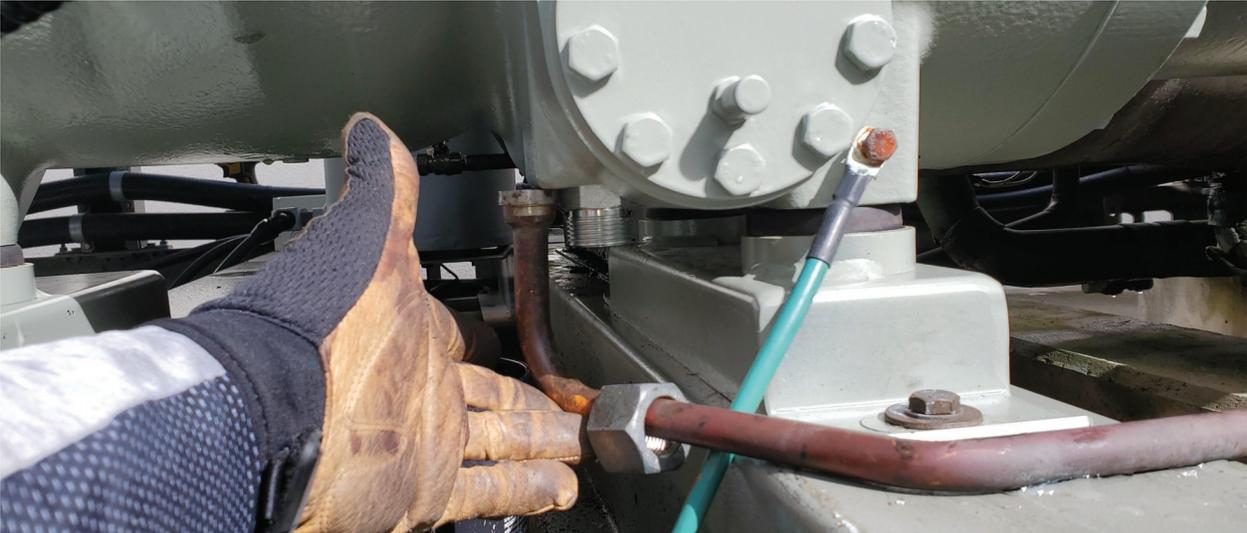
Figure 18. Fitting installation for suction transducer in the suction line
