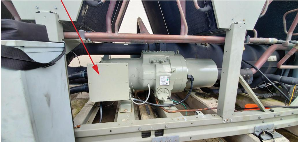
**Figure 12. Cartridge heater location**
