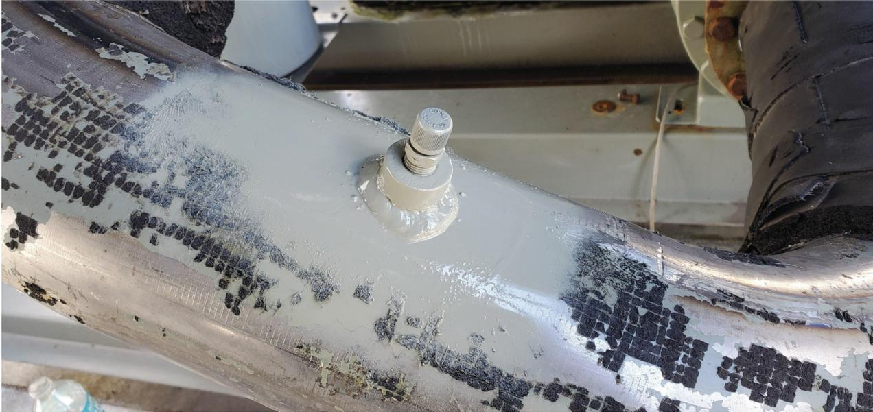
**Figure 22. Install existing suction transducer**
