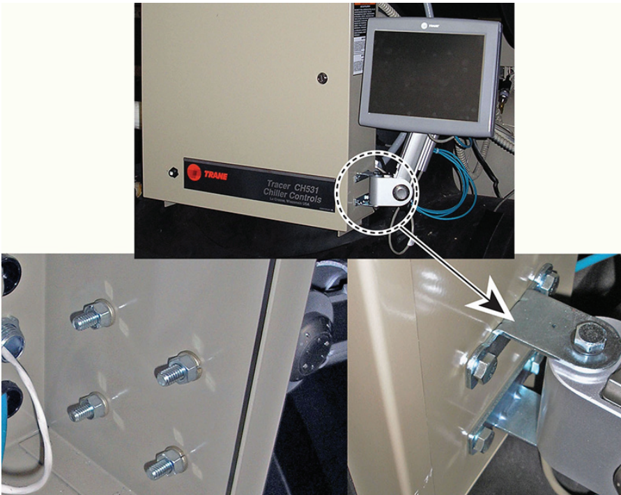
Figure 7. Bolting display arm to the panel
