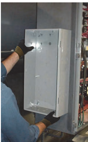
Figure 50. Mounting starter sub-box
