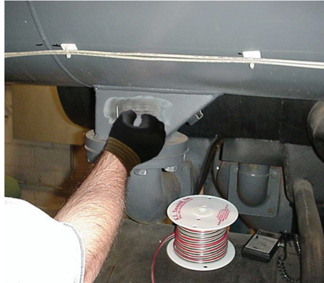
Figure 12. Sensor mounting with Armaflex insulation
