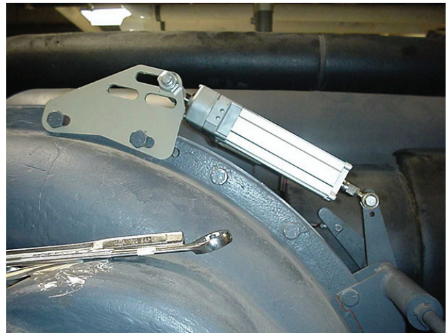
Figure 14. Installed stepper IGV actuator
