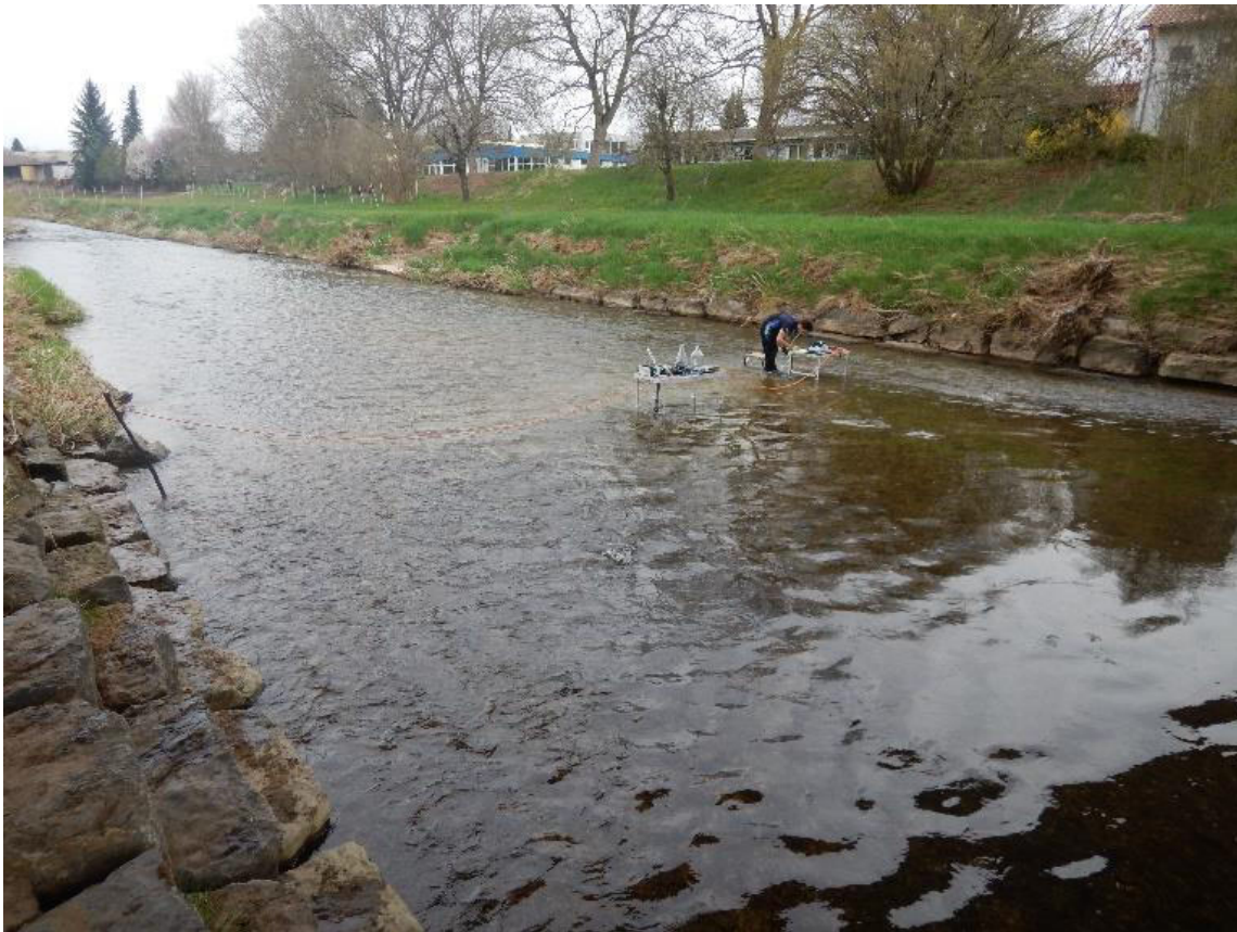
Figure 4.16: Image of River Rems facing downstream direction including measuring set up for Rems 1 and Rems 2.
