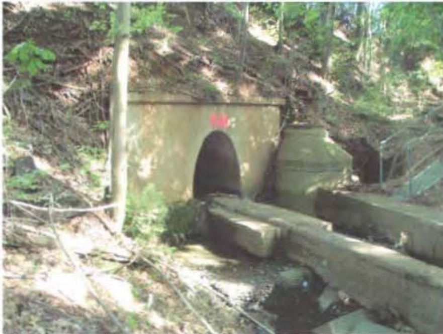
Photo 3: Douglas Battery storm water outfall at railroad on west side of property.
