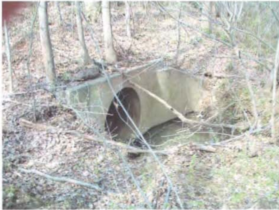
Photo 5: Storm water culvert entrance beneath Starlight Dr.
