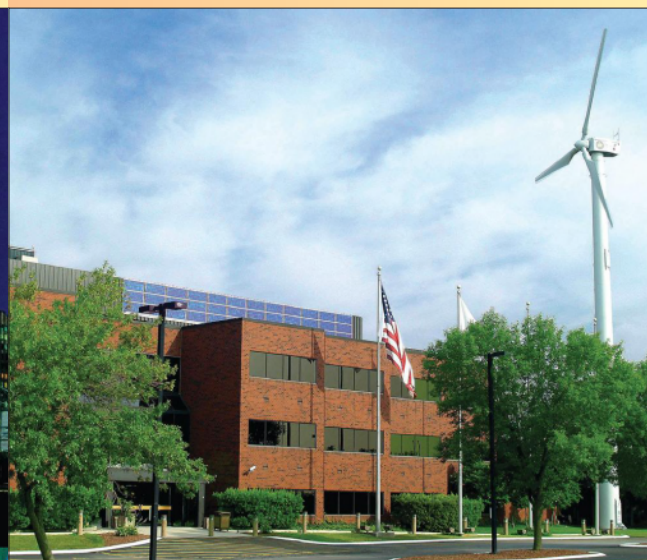
JATC Training Center/Wind Turbine, Boston, MA
