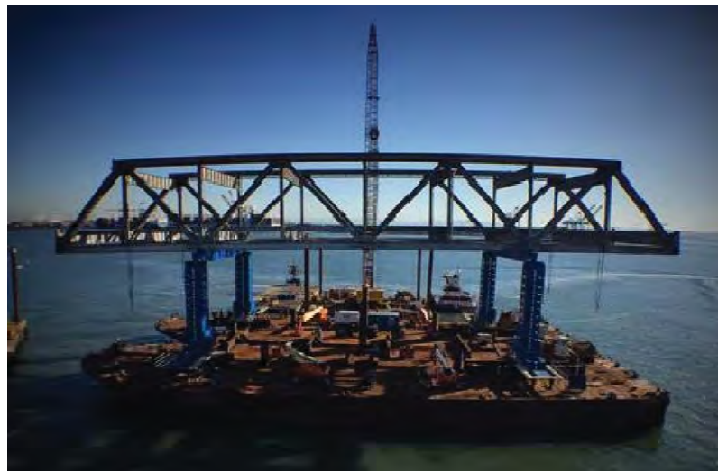
Figure 4 - In-Tact Truss Transport
