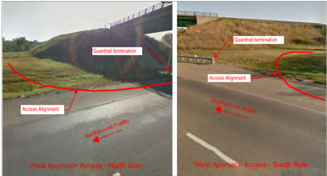
Figure 18-4. West Approach Access
