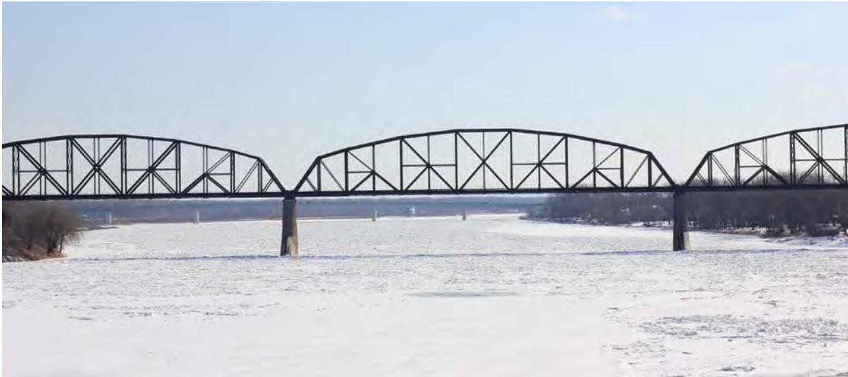
Figure 13: Bridge 196.6 Looking South from Grant Marsh Bridge
