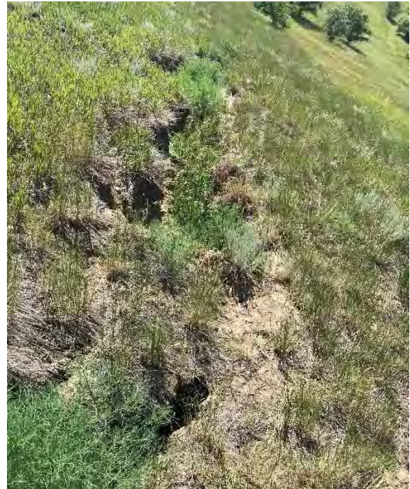
Erosional Features Along Slope
