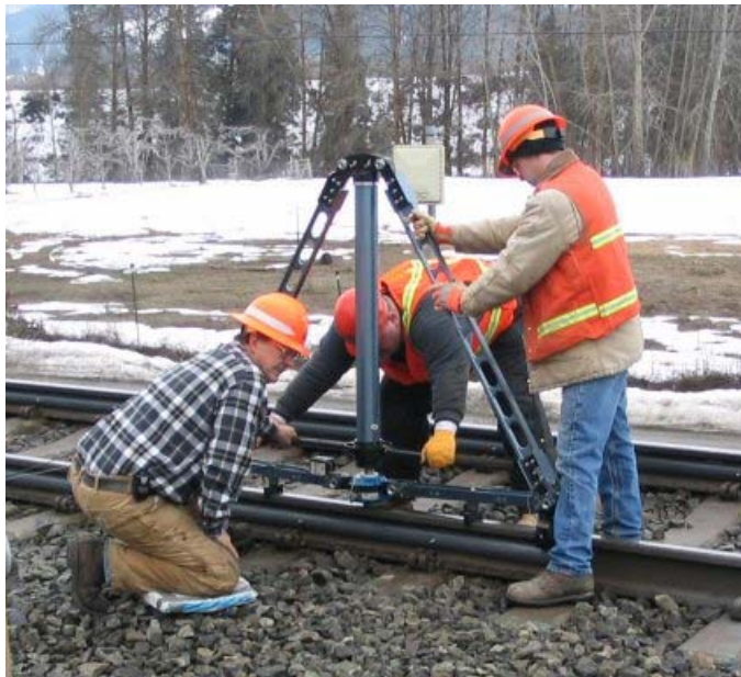
Figure 10.32 Applying force to the rail
