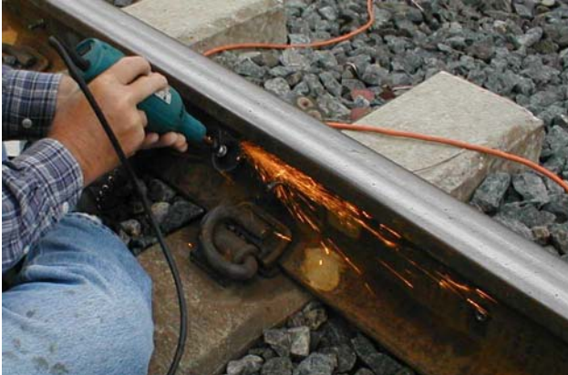
Figure 11.11 Grinding the rail.
