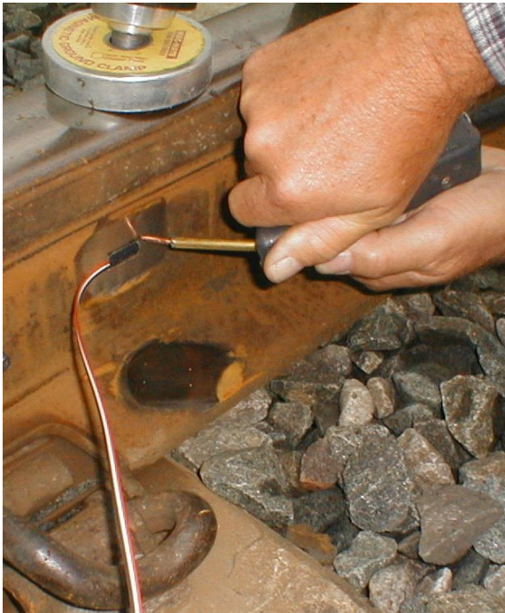
Figure 11.12. Welding the metal coupon.
