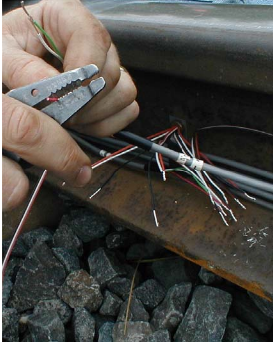
Figure 11.17. Stripping the leads.
