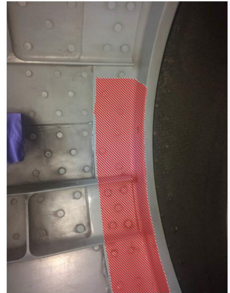
Dye-penetrant inspection of the junction frame
