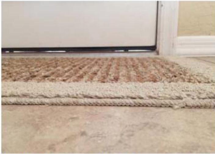
Fig. 1. This locked door is wide open to pests! (Note gaps under door).
