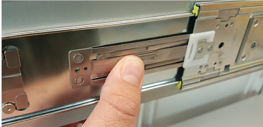
Figure 165: Inner Rail Safety Latch Release
