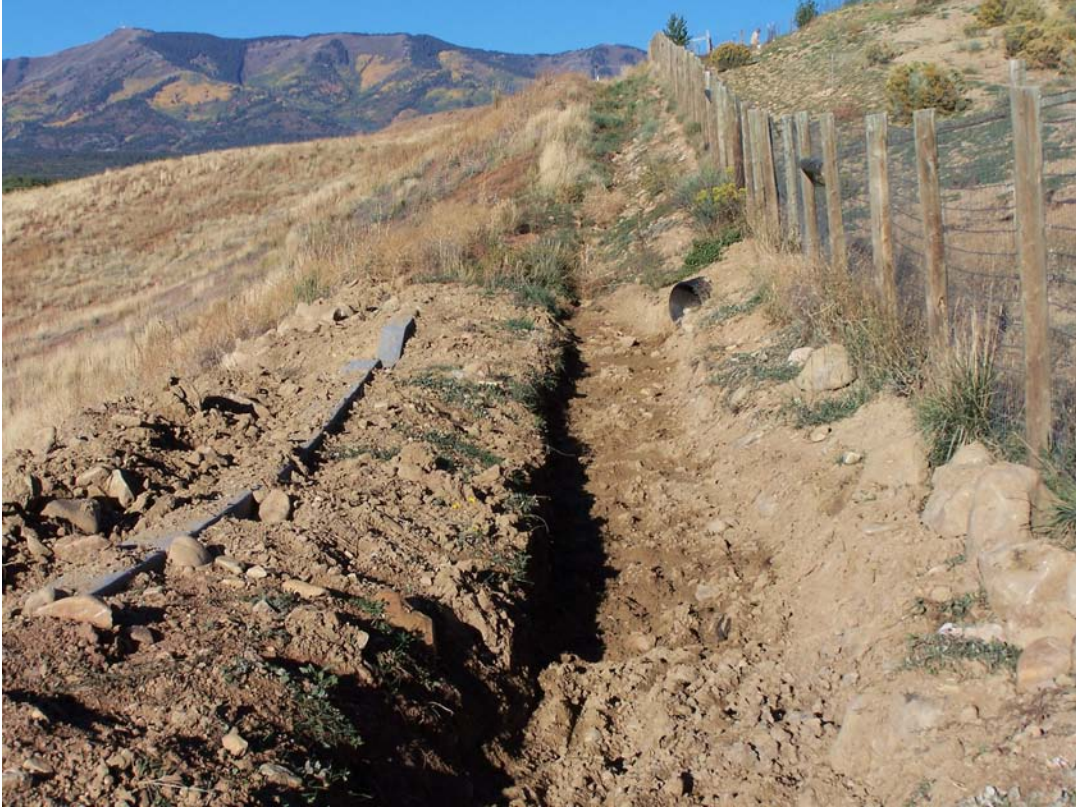
MNT 9/2005. PL-11. Trench and concrete structure below Frost Property culvert.
