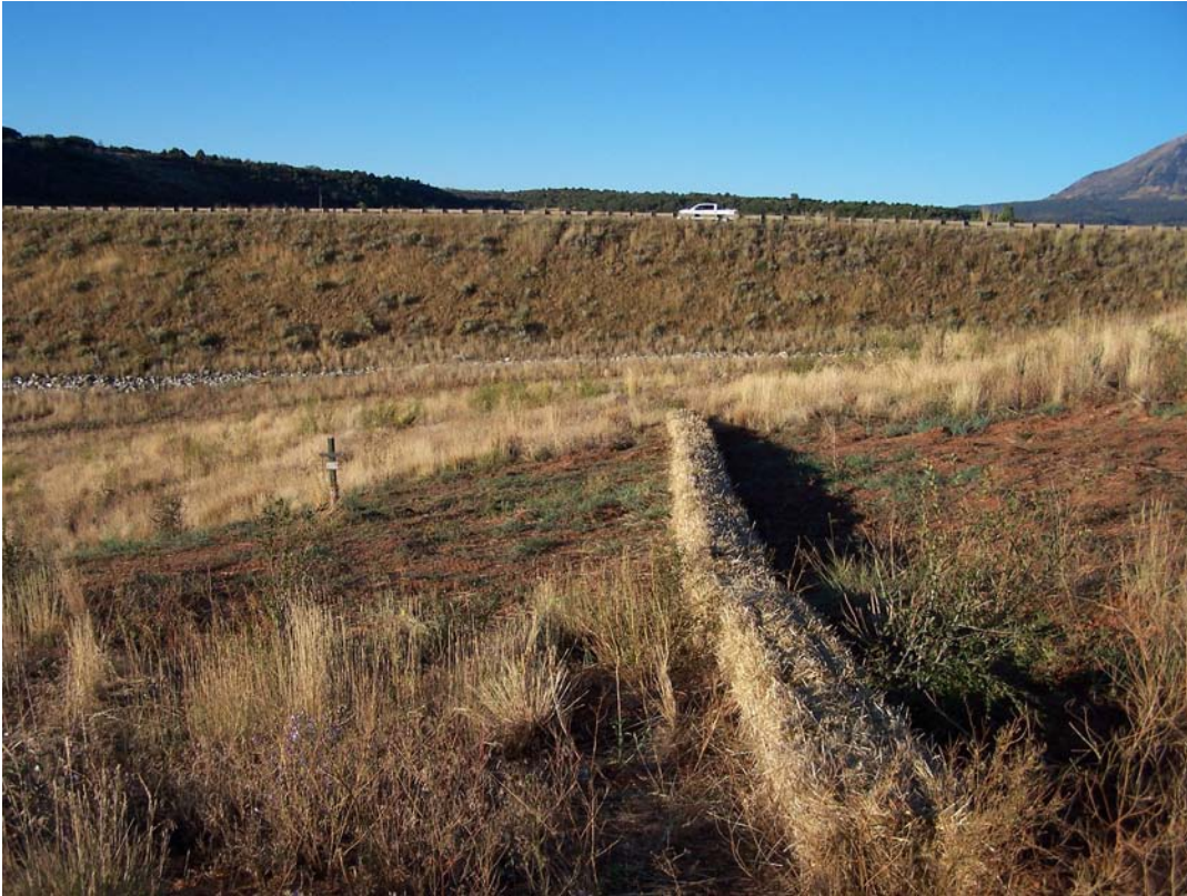
MNT 9/2005. PL-13. Straw Bales controlling erosion west of Goodknight Spring.
