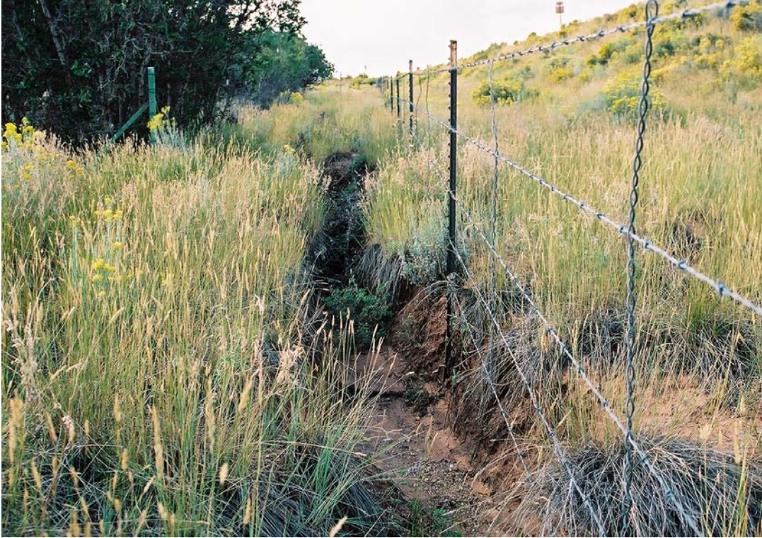
MNT 9/2005. PL-1. Gully erosion near perimeter sign P1.
