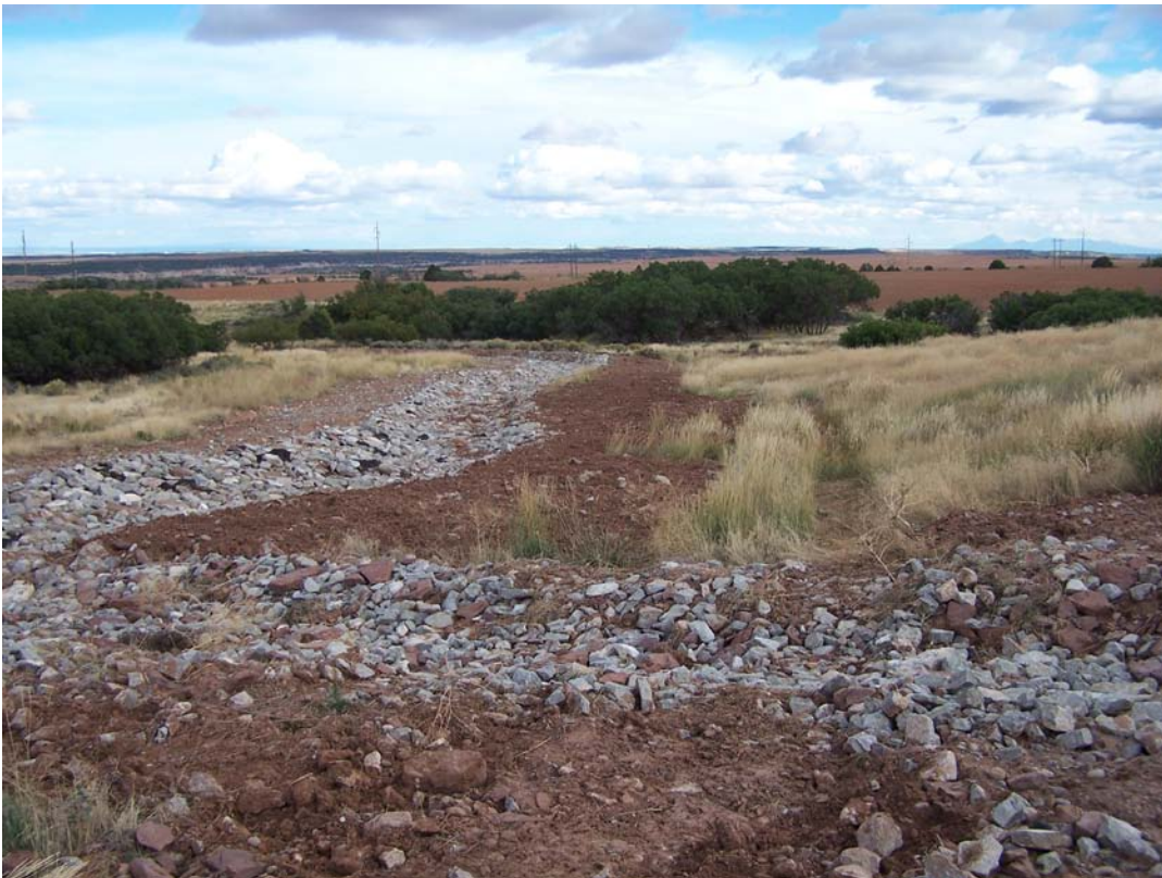
MNT 9/2005. PL-8. Reconstructed channel leading to Sediment Pond C.
