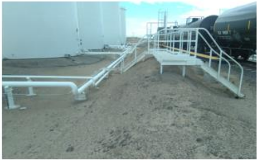
Existing fuel storage tanks to remain
