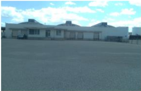
Existing building to be removed
