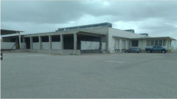
Existing building to be removed
