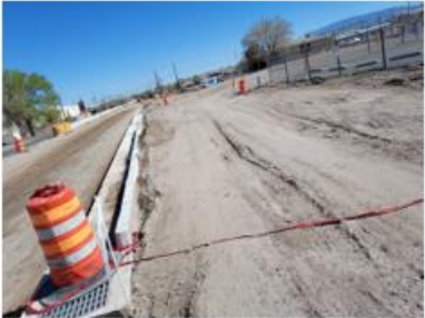
Recent roadway work on Broadway adjacent to site
