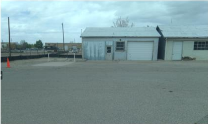
Existing building to be removed
