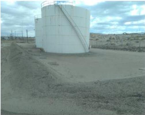
Existing fuel storage tanks to be removed
