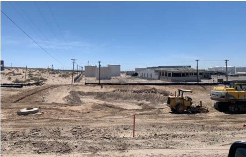
Municipal Drainage pond under construction
