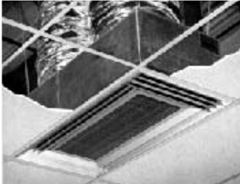
LIGHT COMMERCIAL "T" BAR CEILING
