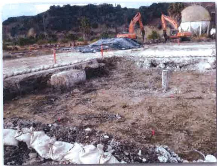
Typical Under Slab Samples (Vicinity of Grid I-L/20-24; Also Note Sumps -06 & -07 )
