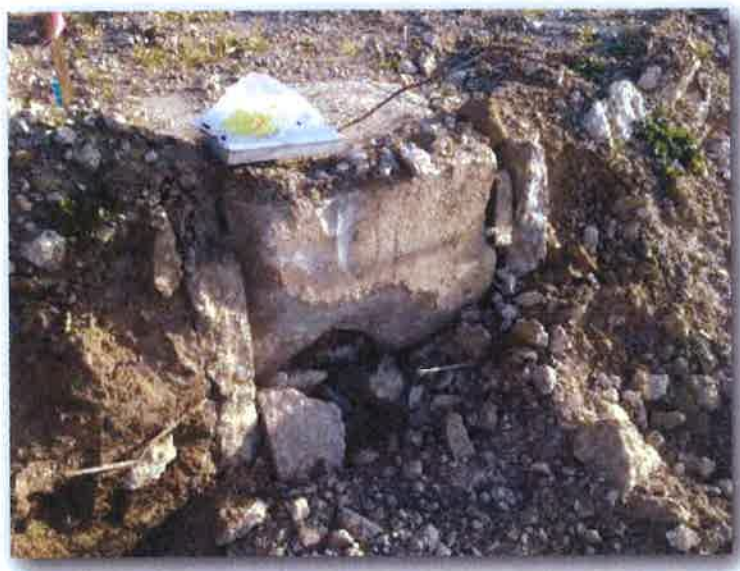
Concrete-Filled Sump-01 During Removal
