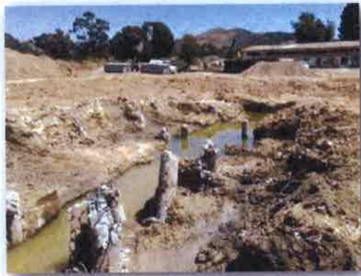
Excavation and Benching After Round 5 Excavation (Looking East)
