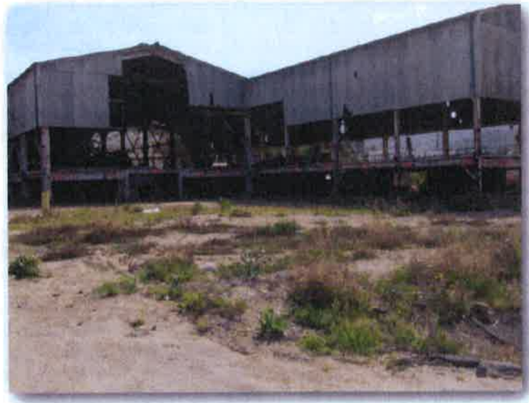
Former Compressor Building
