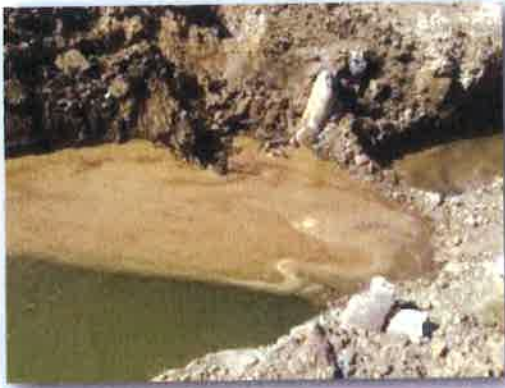
Hydrocarbon Product After Round 4 Excavation (Vicinity of IJ19.5)
