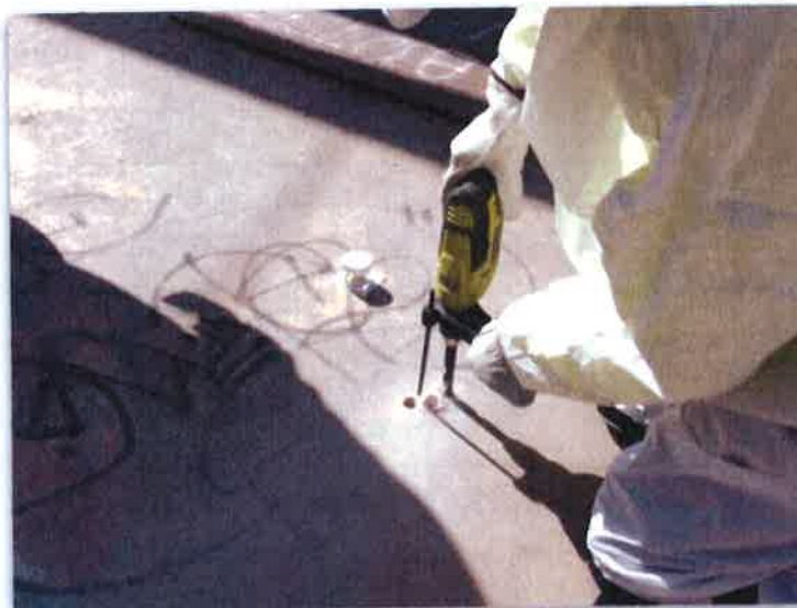
Concrete Hammer Drill Sampling
