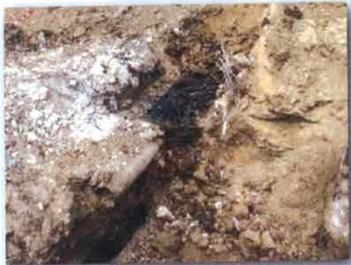
FNDL PIPE Prior to Round 2 Excavation (Vicinity of IJ18.5)
