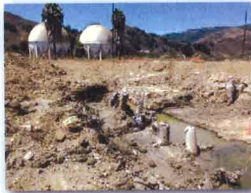
Excavation and Benching After Round 5 Excavation (Looking West)
