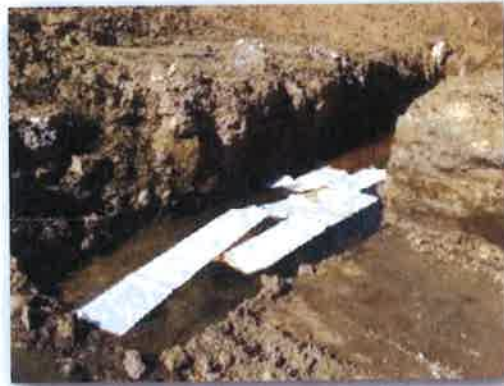
Sorbent Pads Used After Round 4 Excavation
