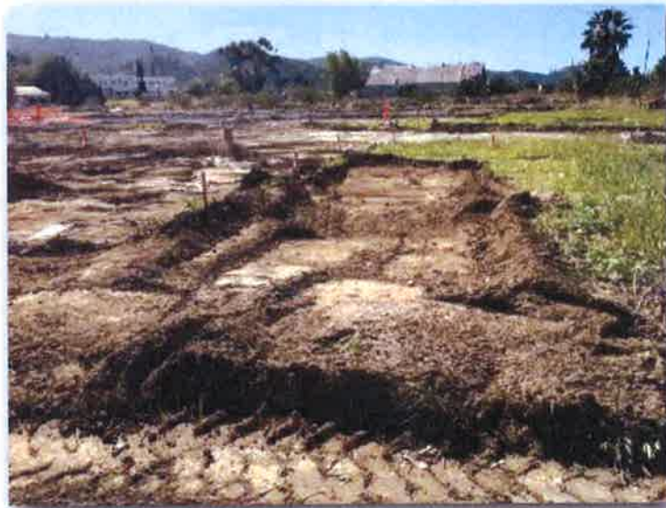
Pb Re-Excavation In-Progress
