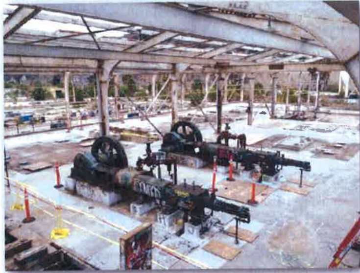
Compressor Building Floor Deck (Note remaining compressors)
