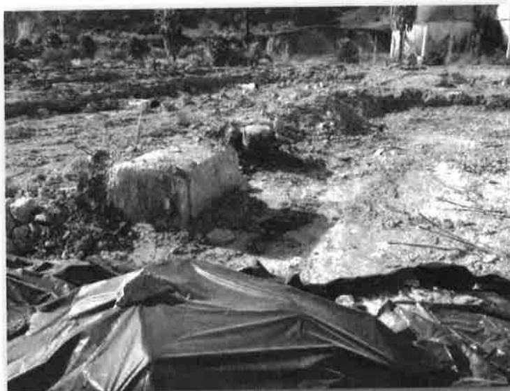
Sump-07 (foreground) and Sump-06 (drums) During Round One (Note staining in adjacent soil)
