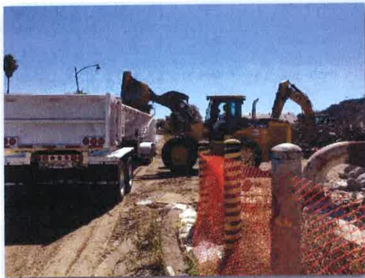
Truck Loading Operations
