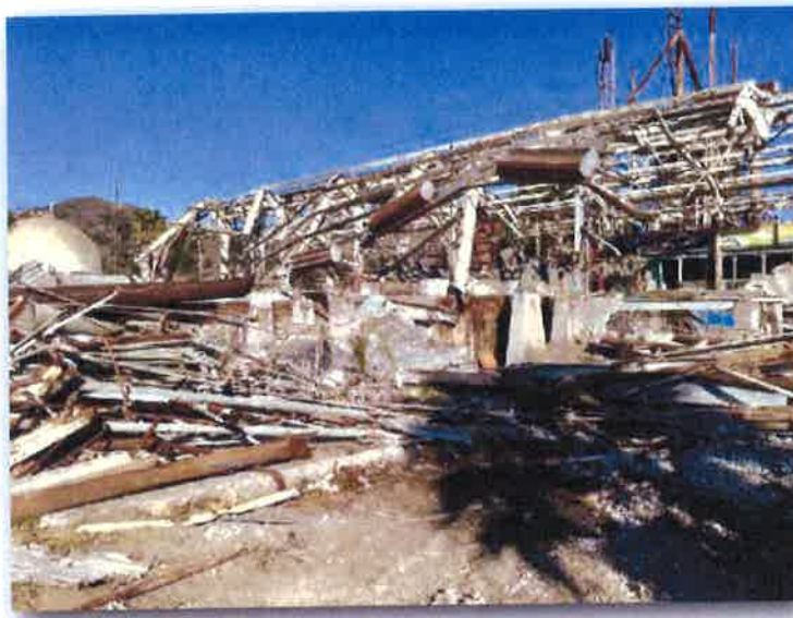
Compressor Building Demolition
