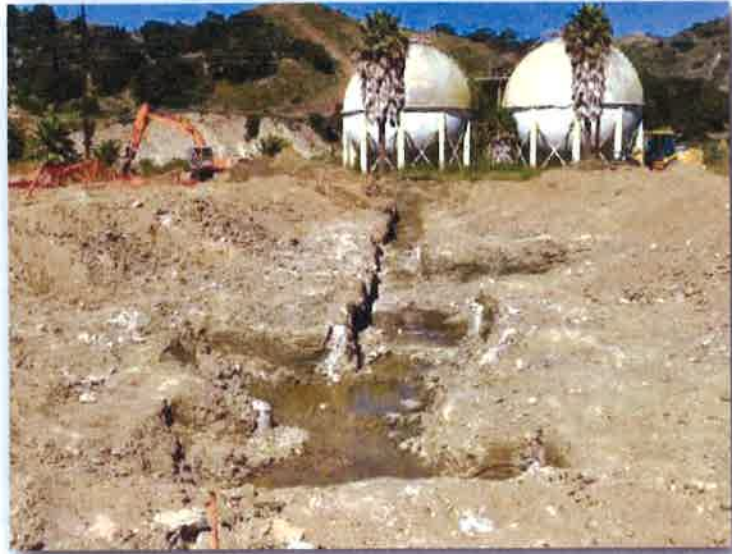
Shallow Groundwater in the Round 3 Excavation (Vicinity of Rows IJ and JK)
