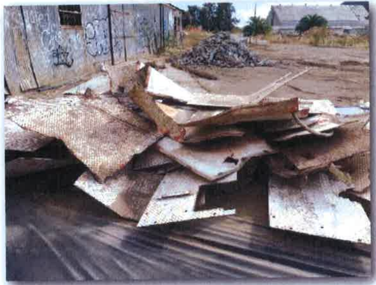
Painted Steel Diamond Plate Staged for Disposal
