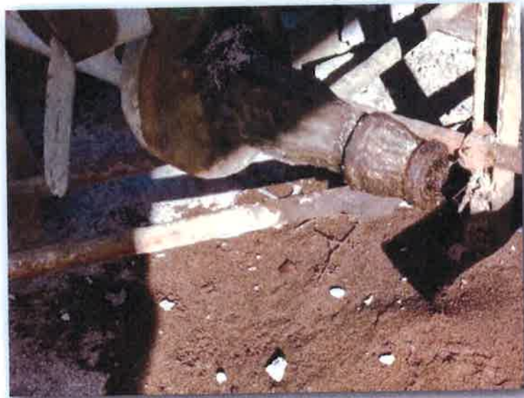
Suspect Pipe and Sorbent
