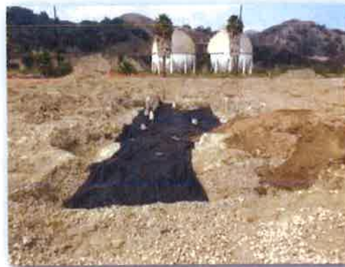
Geotextile Fabric Over Gravel
