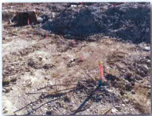
Oil-Stained Soil Encountered During Initial Under Slab Sampling
