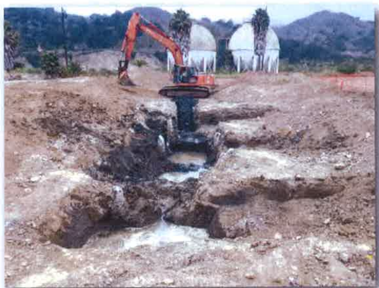
Round Four Excavation
