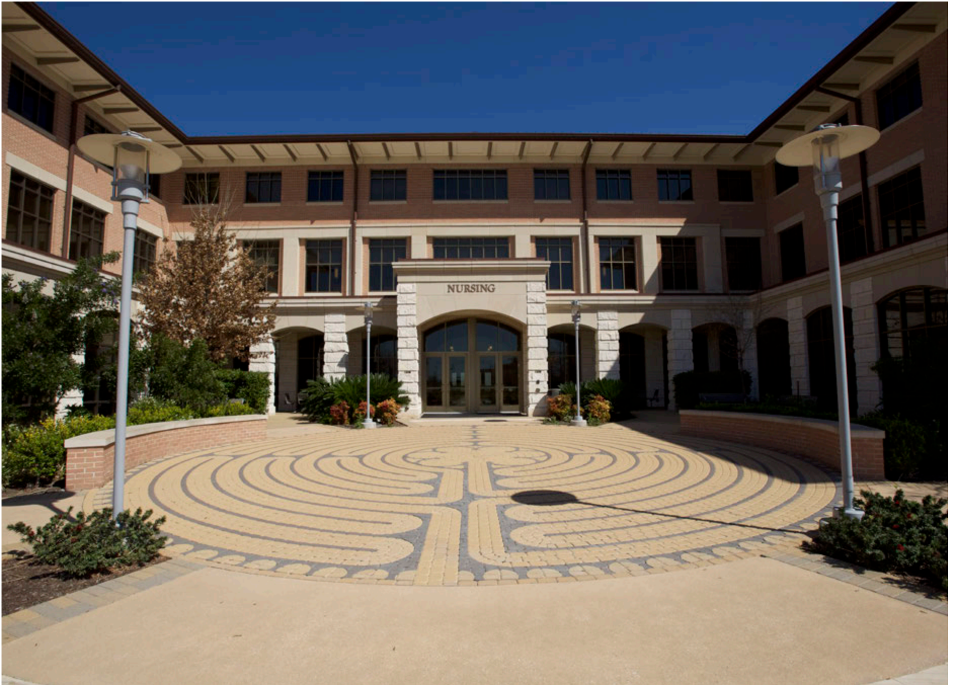
NURSING BUILDING, ROUND ROCK CAMPUS
