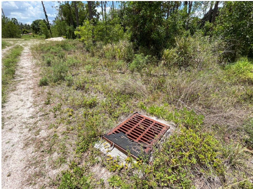
Photo 5: Typical view of storm drain from previous development. View is west.
