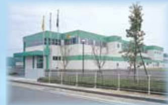
Mie Plant (TA & IT Plant)
