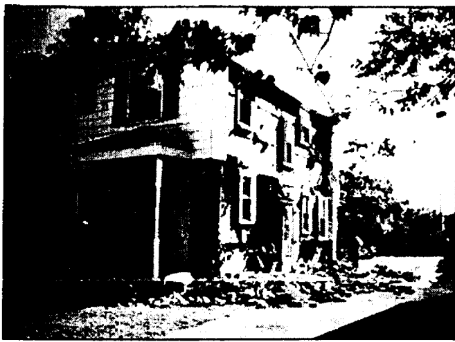
This house on Moross is being prepared for the day, when it will be placed on a flatbed truck and moved to a lot in the Woods.
