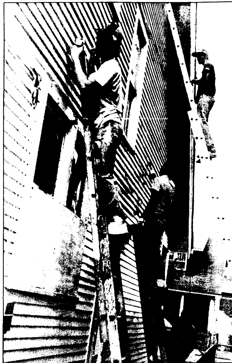
Ben Meyer, 17, of Sioux Center, Iowa, adult supervisor Daryl Baar of Sioux Falls, S.D. and Troy Prinsen, 17, of Sioux Center, Iowa, prepare a house for a new coat of paint.
