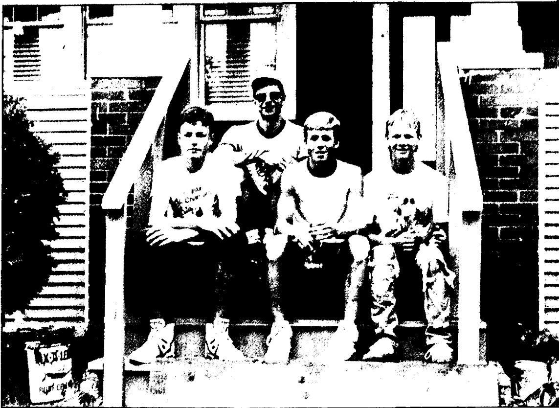
Trent Prins, 15, of Edgerton, Minn., Steve Crull, of Sioux Center, Iowa, Jeremy VanEssen, 15, of Edgerton and Steve Westra, 16, of Sioux Center, take a rain break and a rest on the front porch of a house they're painting.
