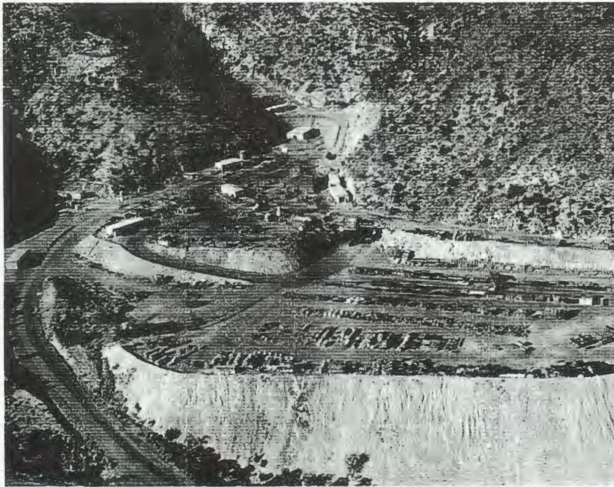
■ Figure 2. Aerial view of the N-Tunnel entrance and associated staging area.
