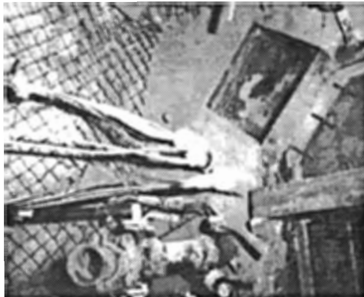
Figure 15 . Pre-event photograph of the end of the grouted area of tunnel showing pipes and other things that could have damaged pressure lines.
