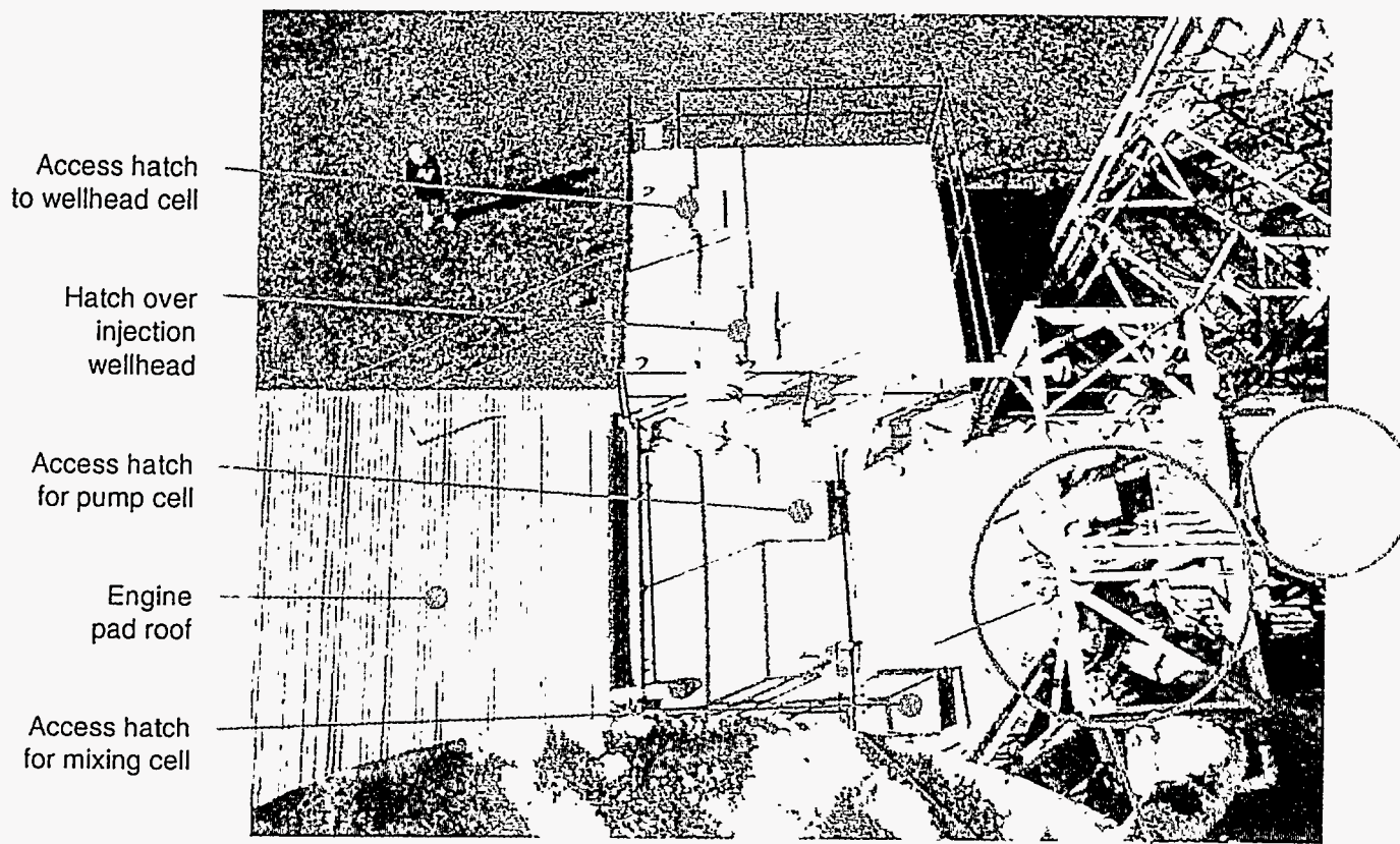
Fig. 2.7a. Roof of Building 7852 as seen from top of Bin 4.
