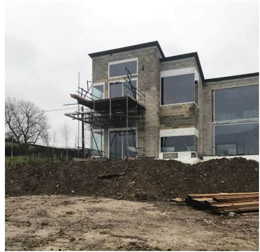
(Rear of as constructed replacement Dwelling)
