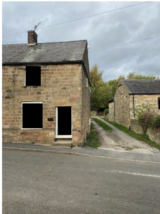
Photo 1: Southern elevation of Buxton House fronting Main Street showing the windows to be replaced and the private access track / PROW
