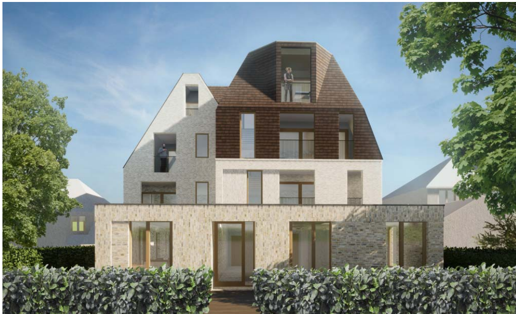
Rear elevation showing single storey rear projection
