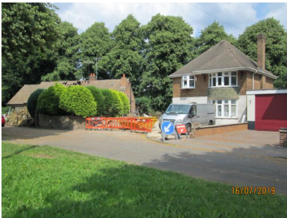
Existing bungalow and dwelling at 3 Queens Road East.
