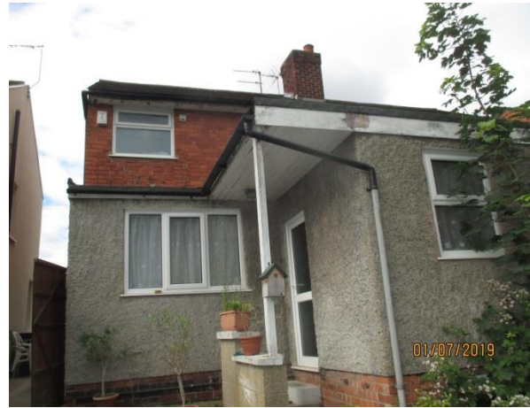
Existing rear extension
