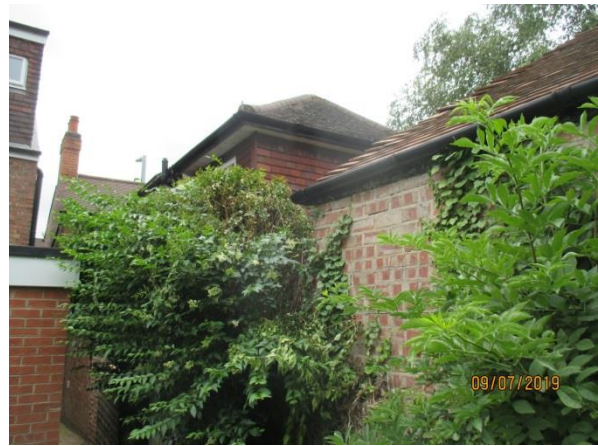
Boundary to 26 Lower Road
