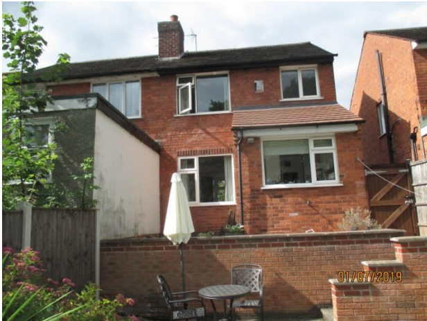
Rear elevation of 76, showing the existing extension to 74 to the left
