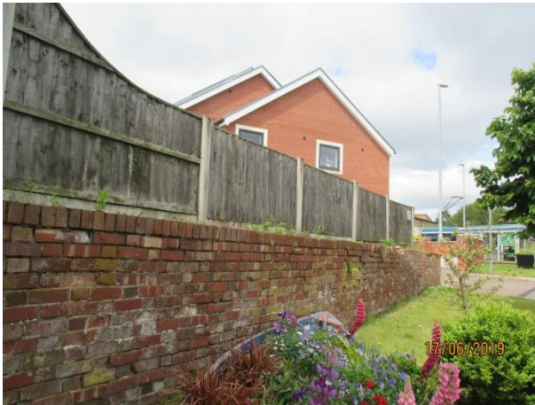
Retaining wall to car park of Flewitt House, taken from the grounds of the resource centre
