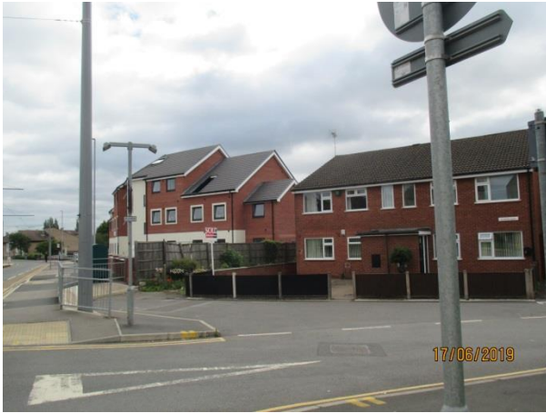
Flewitt House, to the left, with Churston Court to the right
