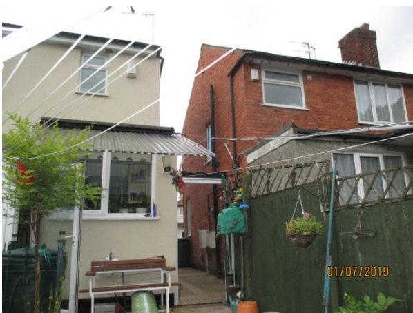
Rear elevation of 72 to the left
