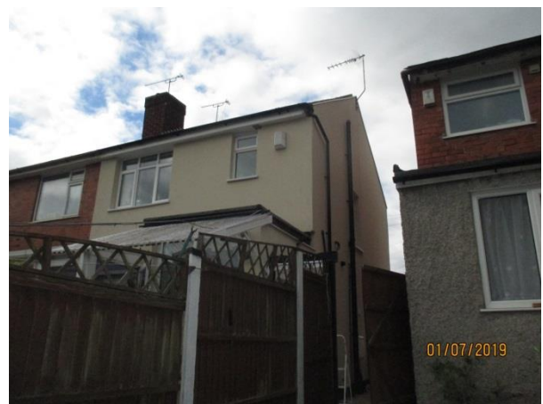
Rear elevation of 72 from the application site
