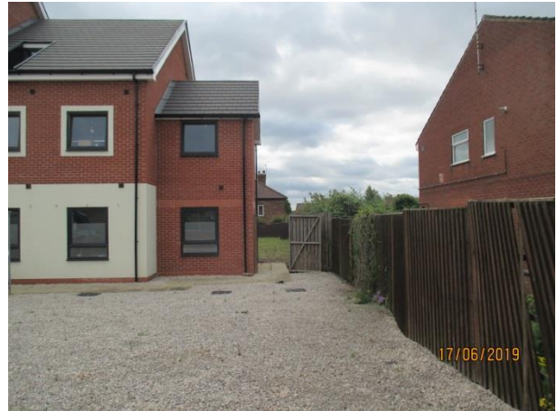
Gap between Flewitt House and Churston Court
