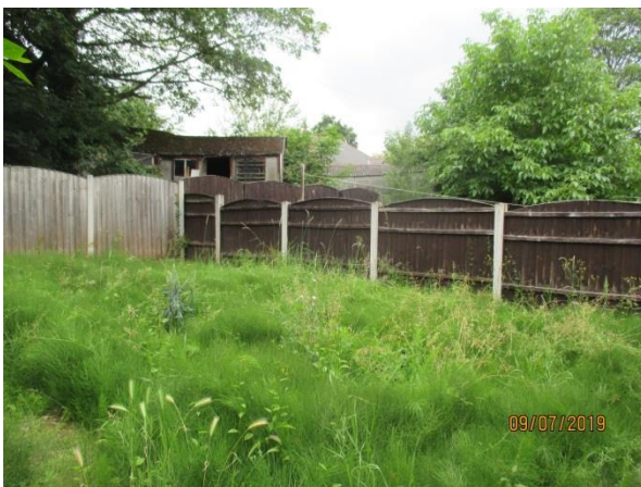
Boundary to 22 Lower Road
