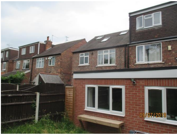
Rear elevation with 22 Lower Road to the left. Room to be converted to the left side of the rear extension
