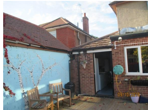
Rear yard, showing garage within 173 Attenborough Lane, forming the south east boundary
