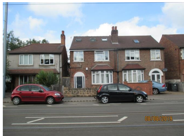
24 Lower Road to the centre, with 22, the attached semi, to the right
