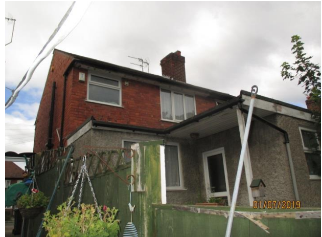
Rear elevation of 74 Peveril Road
