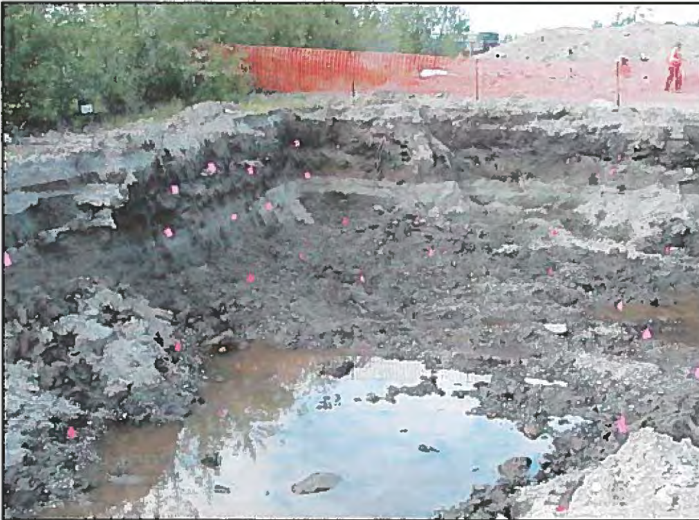
Photograph 11 Final excavation pit 1 viewed NE
