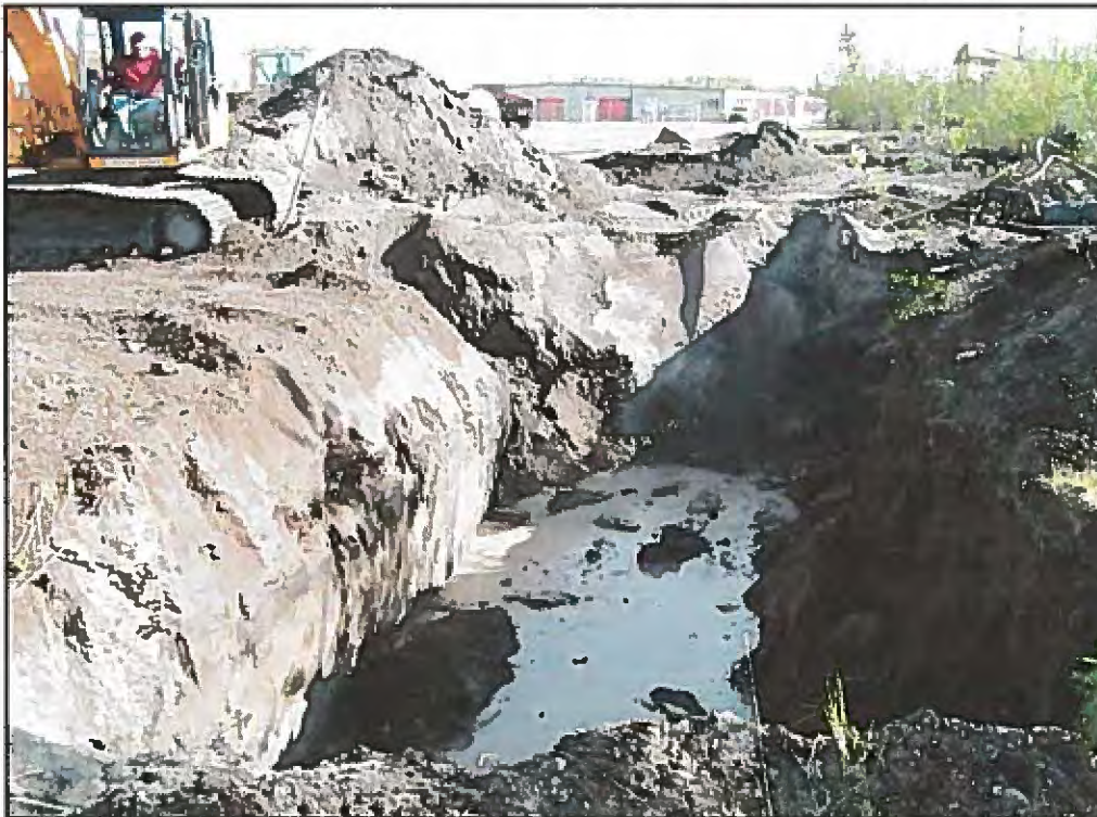
Photograph 7 Final excavation pit 2 viewed SW
