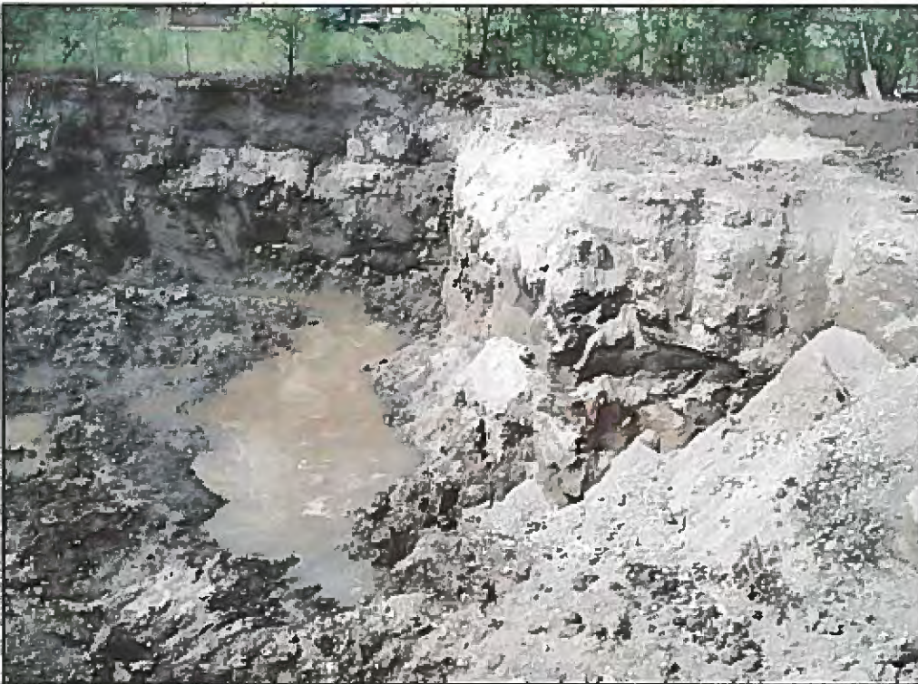
Photograph 5 Excavation pit 2 viewed SW
