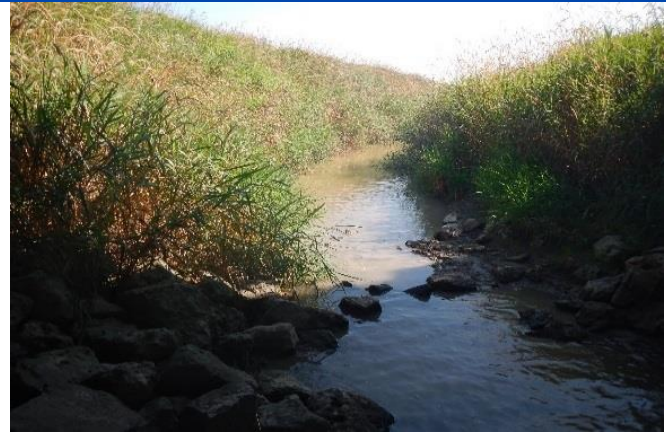
Figure 69 — Platter Creek at Fountain Rd. (RM 5.40).
