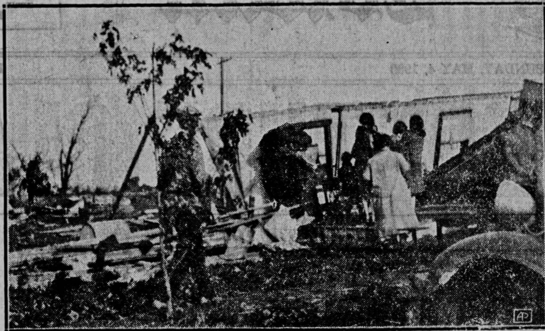
The ruins of what had been a comfortable farm home near Norborne, Mo., are shown above. The storm's force burst apart the walls of this residence but left the piano unharmed. Five persons were killed in and near Norborne and 20 others injured.
