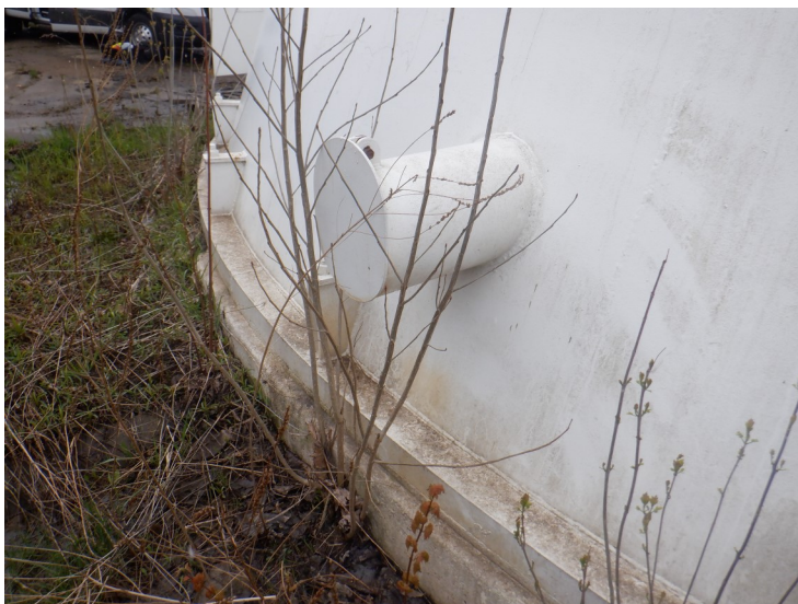
6) The overflow pipe discharges to a concrete splash pad.
