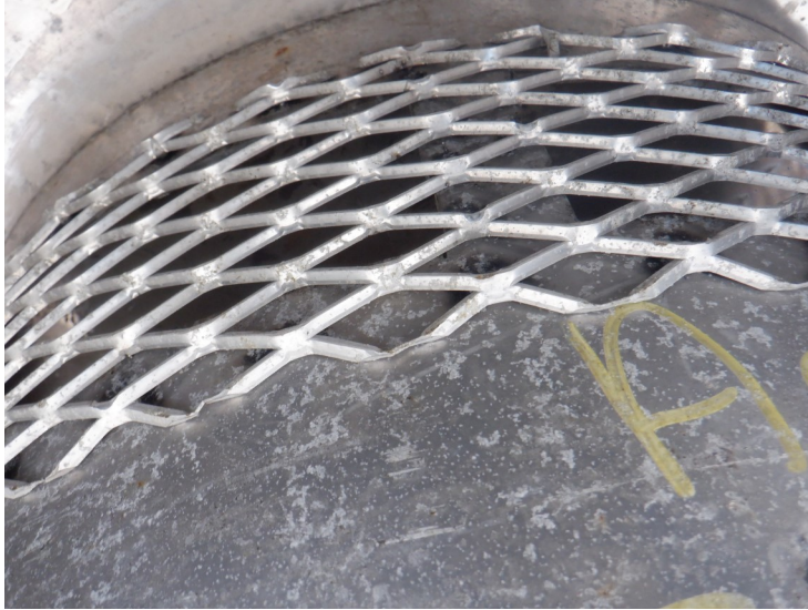
31) The exterior roof vent screen is intact.
