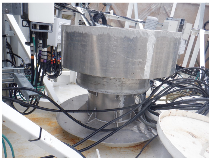
30) The roof vent is in good condition.
