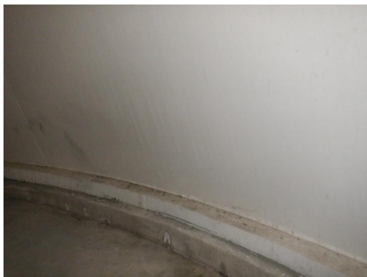
36) The dry interior basebell coating is in good condition overall.
