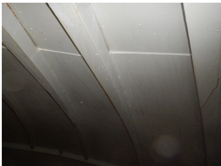
66) The wet interior roof coating is in good condition overall.
