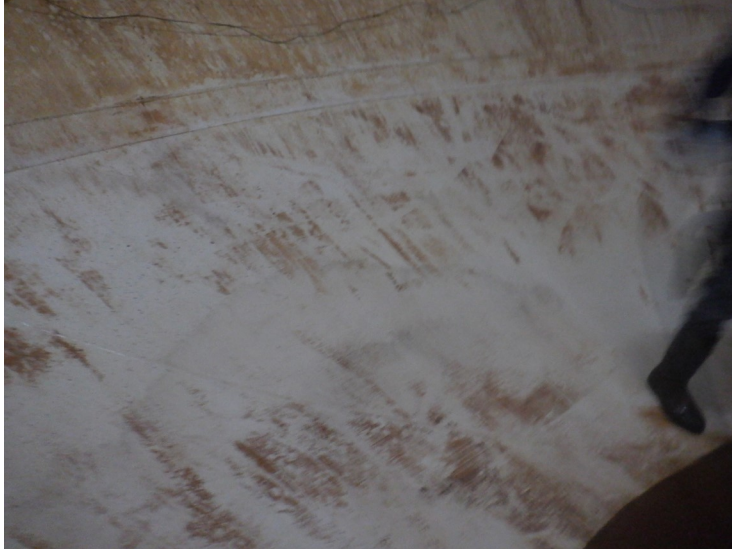
76) There is no significant coating deterioration in the bowl.
