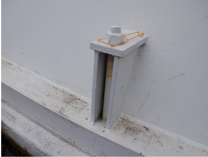
4) The anchor bolts are in good condition.
