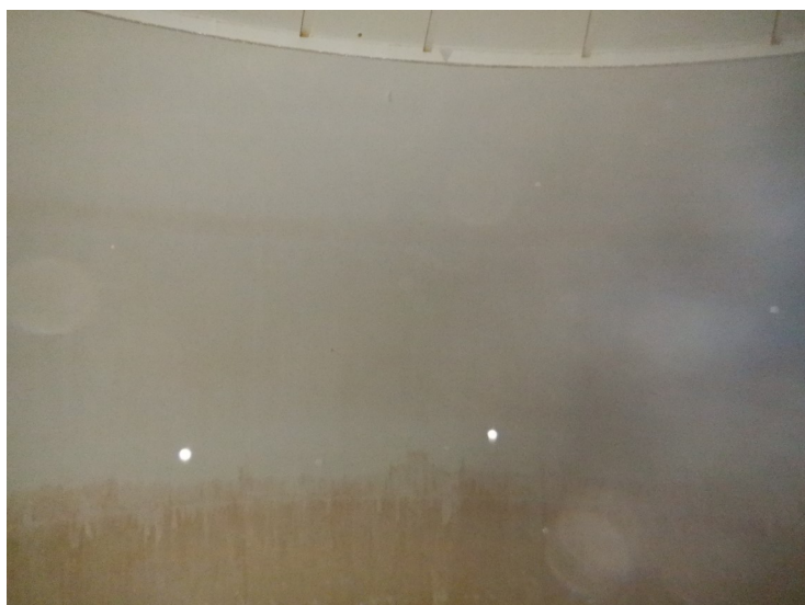
69) There is no significant coating deterioration on the wet interior sidewall.
