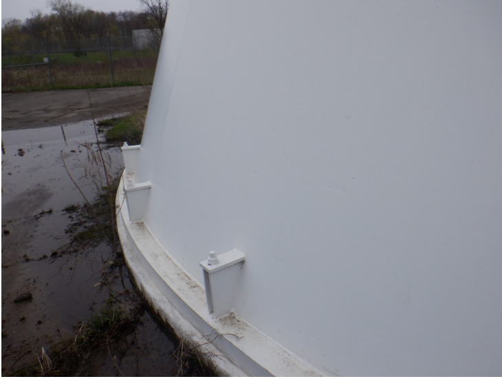
10) The basebell coating is in good condition overall.
