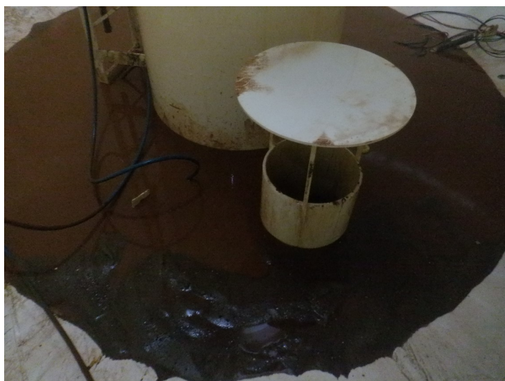
78) There is a deflector plate over the fill/draw pipe in the wet interior.
