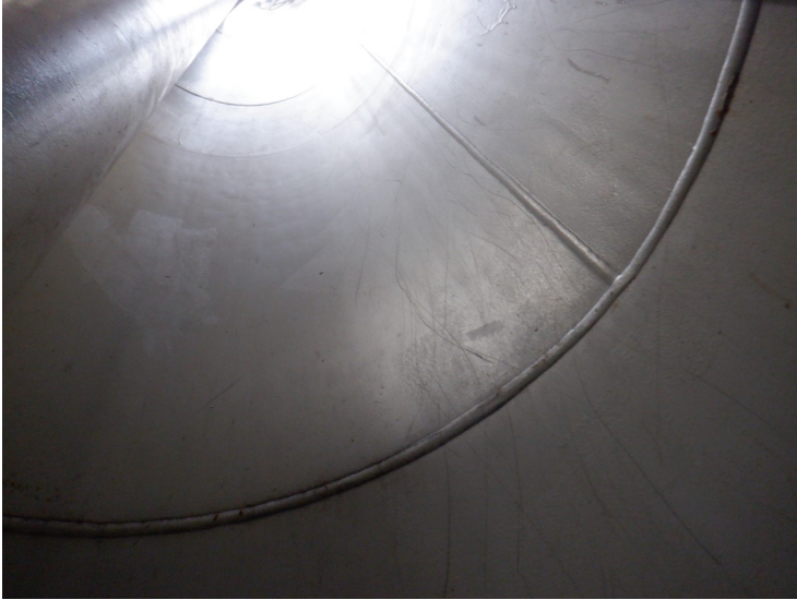
61) The access tube coating is in good condition overall.
