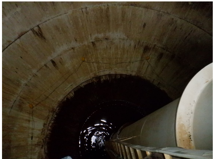
77) The cathodic protection system appears to be in good condition.
