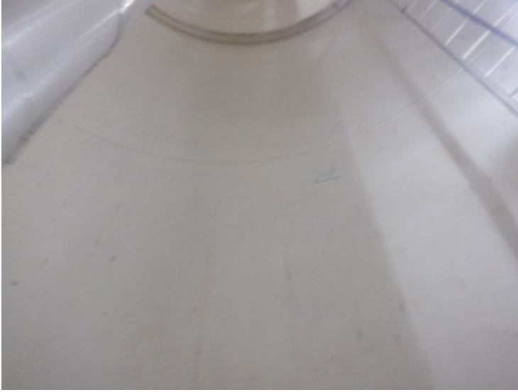
46) The coating in the dry riser is in good condition overall.
