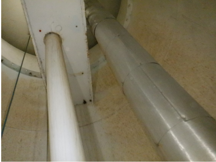
49) The fill/draw pipe insulation and aluminum cover are in good condition.
