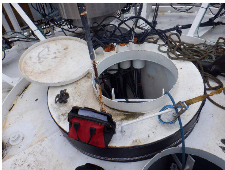
27) There is a handhold at the roof hatches.
