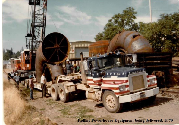
Rollins Powerhouse Equipment being delivered, 1979
